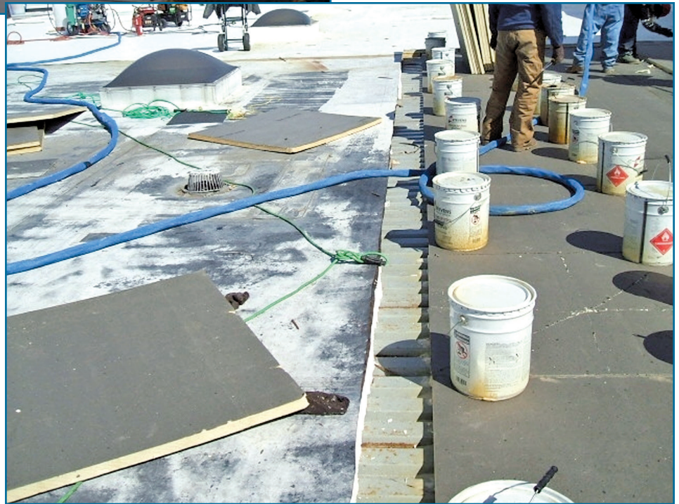
Figure 2 – Old roof system on left; new roof system on right.
