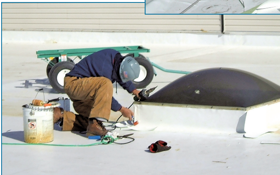
Figure 4 – Roofer performing flashing detail work around skylight.
