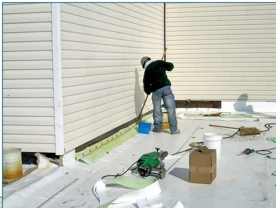
Figure 3 – Roofer performing perimeter flashing detail work.
