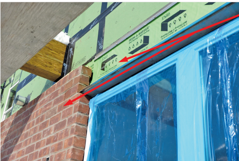
Figure 6 – The masonry subcontractor is also responsible for installing the lintel through-wall flashing. This component can contribute to leaks if defective.
