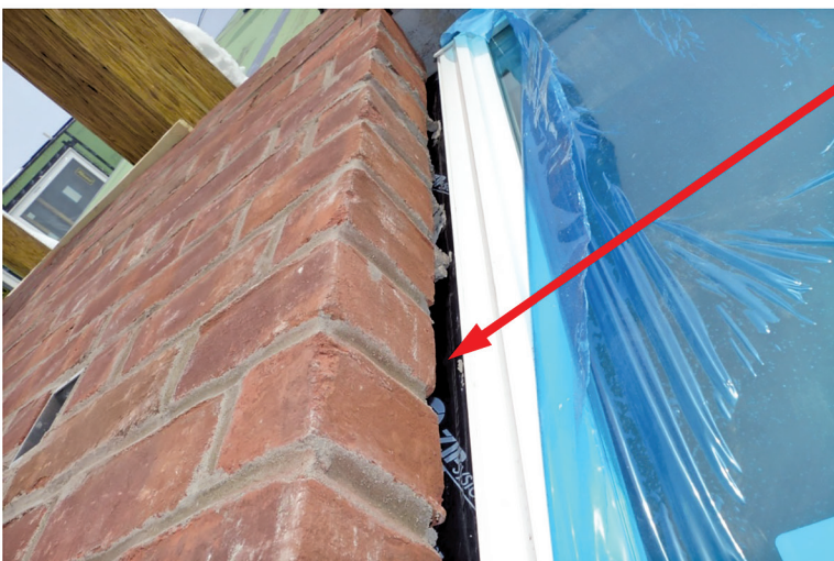
Figure 6 – The masonry subcontractor is also responsible for installing the lintel through-wall flashing. This component can contribute to leaks if defective.
