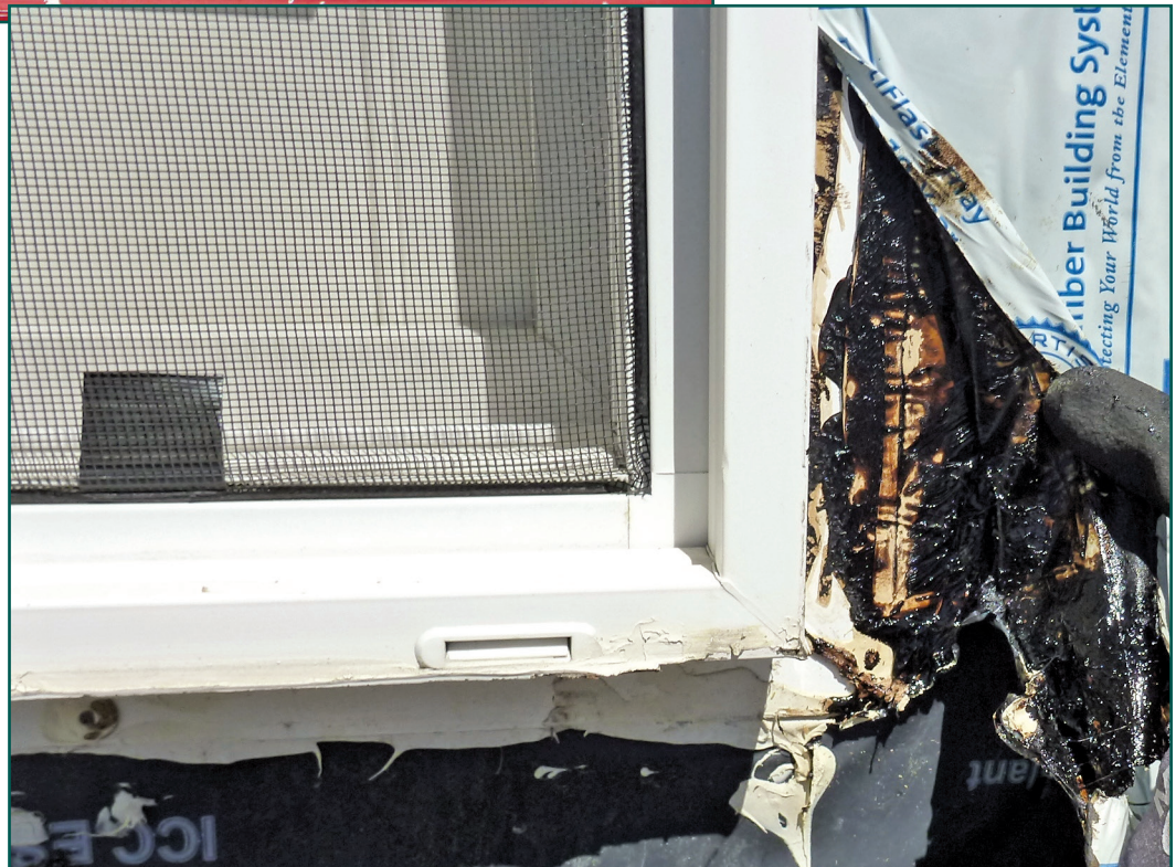
Figure 2 – In 2017, our destructive sampling at a multi-building condominium complex with 3,200 windows confirmed the material degradation that can occur when incompatible flashing/sealing products are integrated within the building enclosure. Only one defense consultant climbed the ladder to document this project-wide condition.
