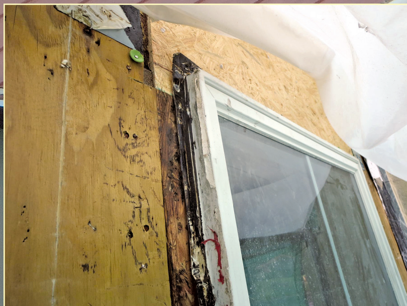
Figure 2 – View of repairs adjacent to an existing window.
