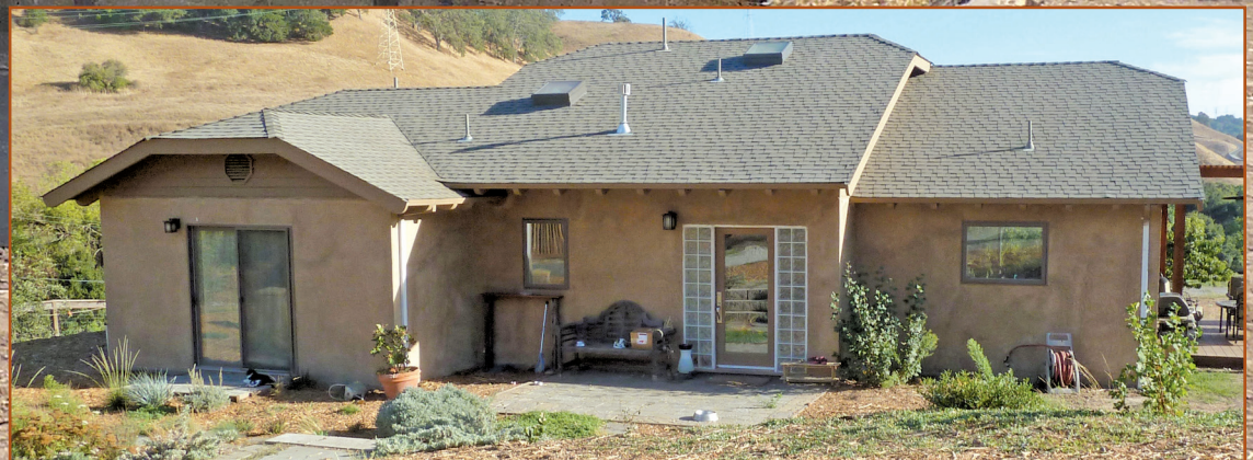
Figure 5 – Completed residence in Martinez, CA, from Figure 4.
