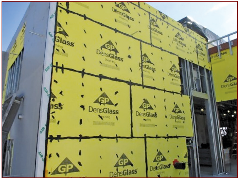
Figure 3 – Pretreatment of sheathing joints and fastener heads.
