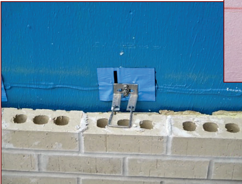
Figure 16 – Cut strip of self-adhered membrane applied on top of fluid-applied air barrier at masonry anchor.
