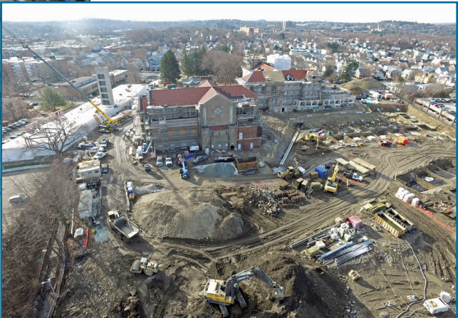
Figure 13 – Construction site audit including 3-D models (orthomosaic) accurately stitched from thousands of photos to annotate and track building changes over time. The aerial image inset was taken at the onset of construction in July of 2018.
