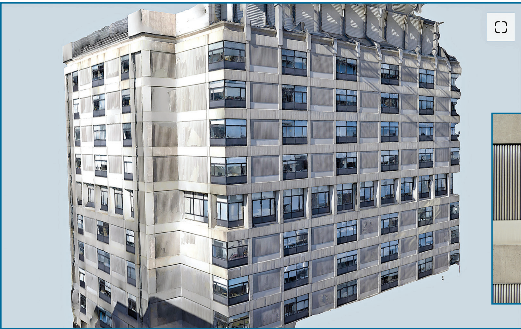
Figure 11 – UAVs are used as tools to render 3-D models of a facade inspection. Interactive software allows the client to access and inspect a building façade one high-resolution image at a time while maintaining a sense of location (native image inset).
