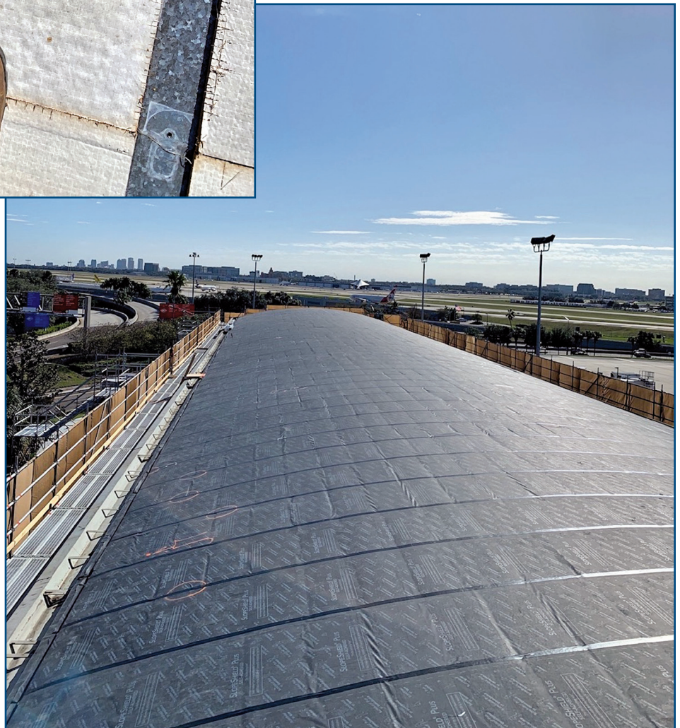
Figure 11 – Installed air barrier at Tampa Airport.
