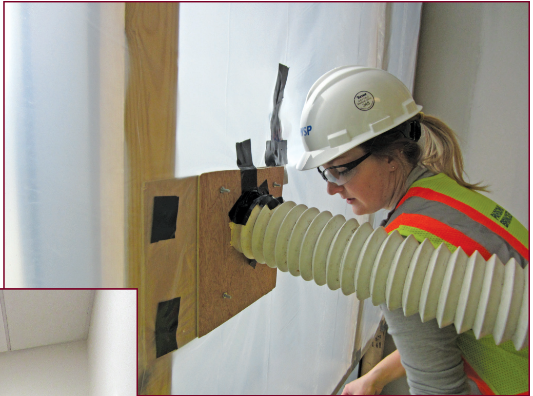
Figure 2 – Observation of water infiltration testing.
