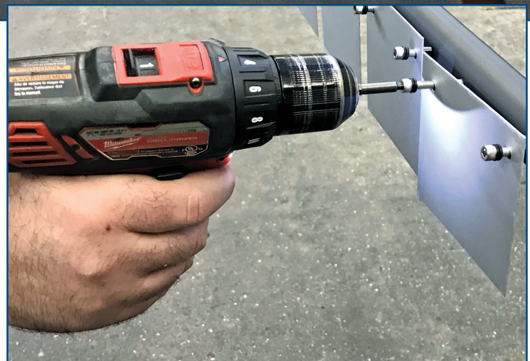
Figure 7 – Pin-mount suspension systems allow the flappers to be removed and replaced without any specialized tools if repair or maintenance is needed on wind-driven kinetic façade systems.
