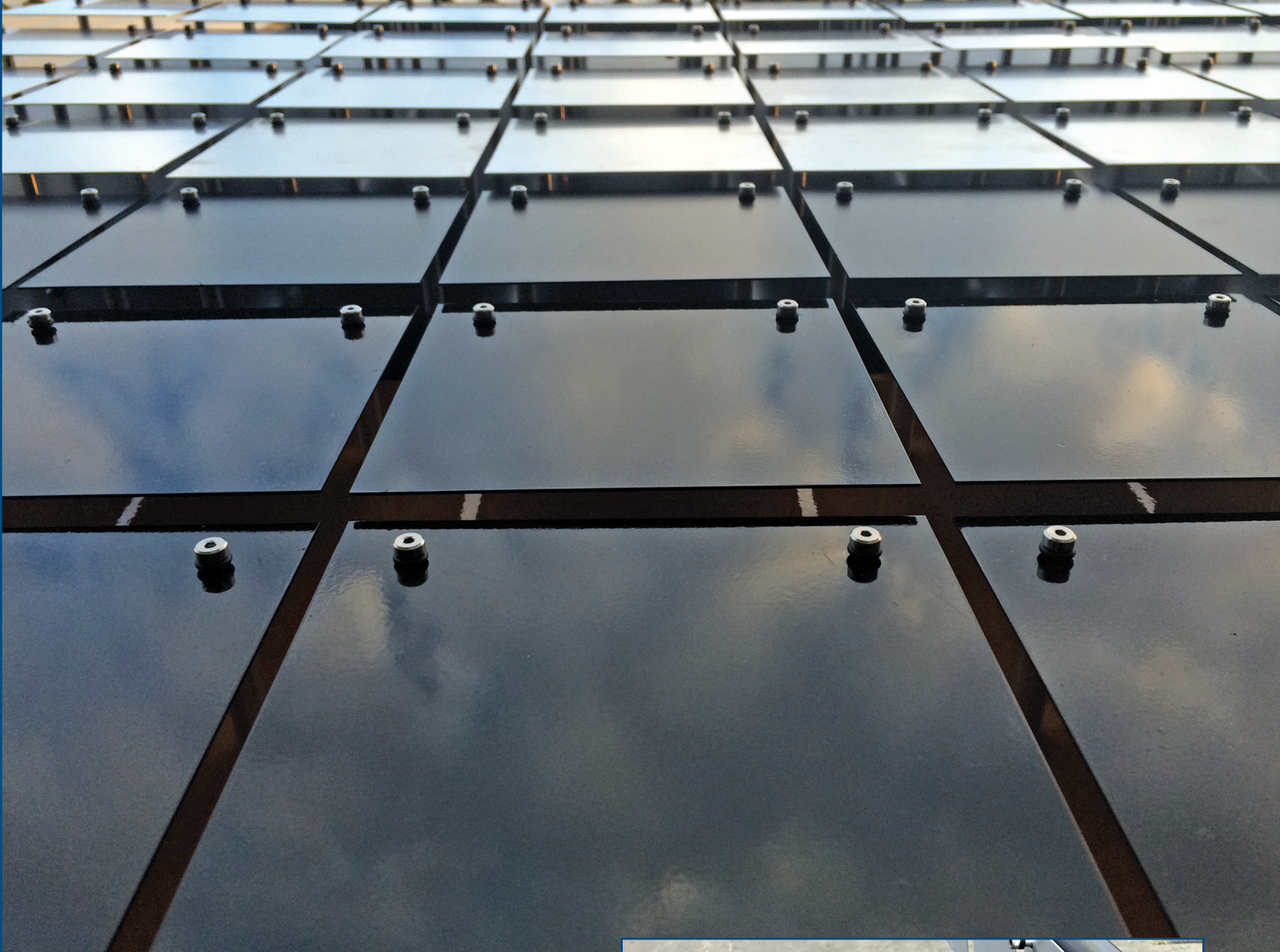
Figure 6 – A pin-mount suspension on a wind-driven kinetic façade system allows the flapper elements to seemingly float in front of the support rungs and side rails as a veil.
