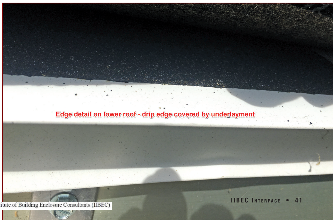
Figure 2 – Picture of underlayment over drip edge.
