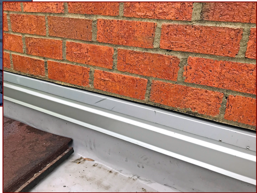
Figure 4 – Through-wall flashing.
