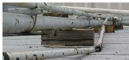
Severe damage to roof and pipe due to the use of wood blocks.
