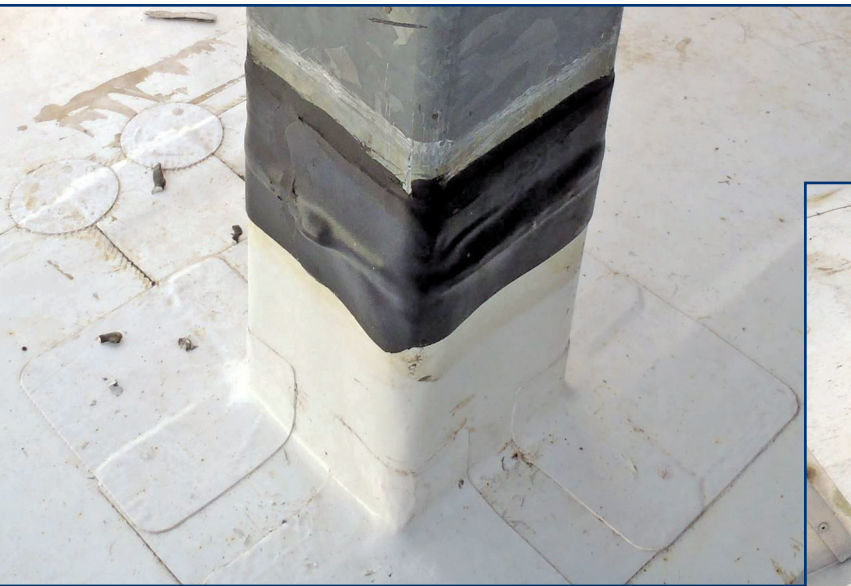
Figure 11a – Elastomeric membrane counterflashing at HSS column.
