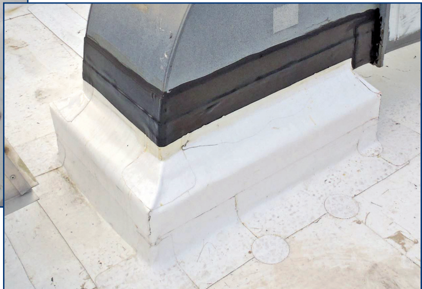
Figure 11b – Elastomeric membrane counterflashing at duct penetration.
