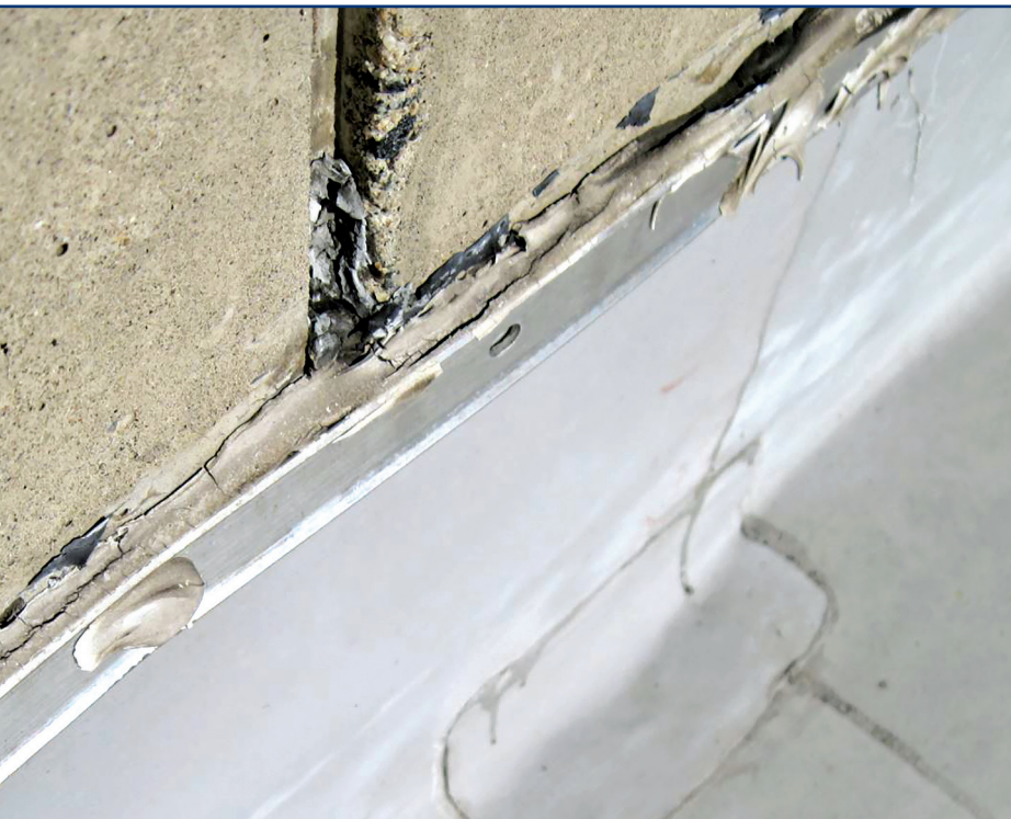
Figure 8 – Vertical joint in precast concrete wall system.
