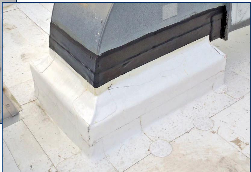
Figure 11b – Elastomeric membrane counterflashing at duct penetration.
