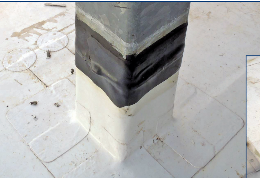
Figure 11a – Elastomeric membrane counterflashing at HSS column.
