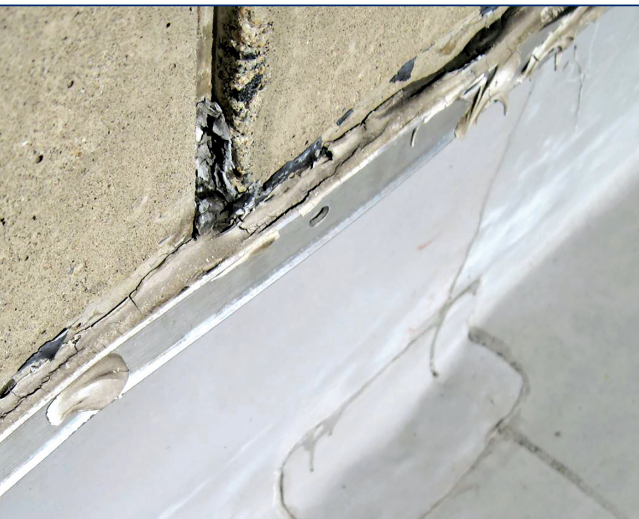
Figure 8 – Vertical joint in precast concrete wall system.
