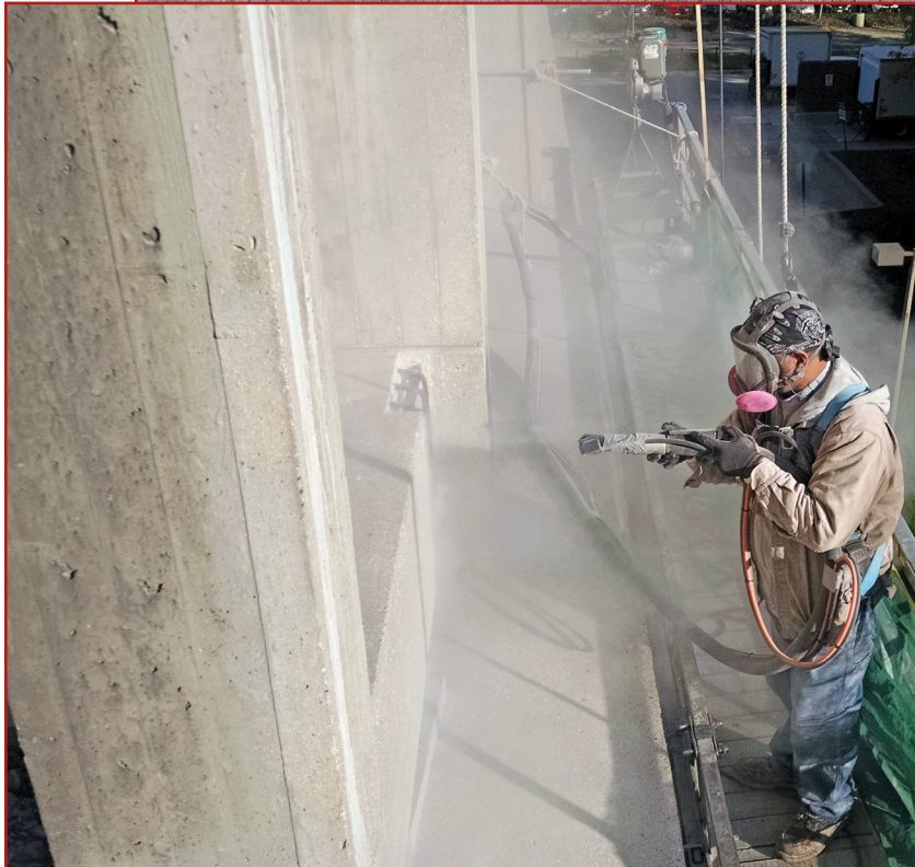
Figure 8 – Soda blasting used during concrete façade cleaning.
