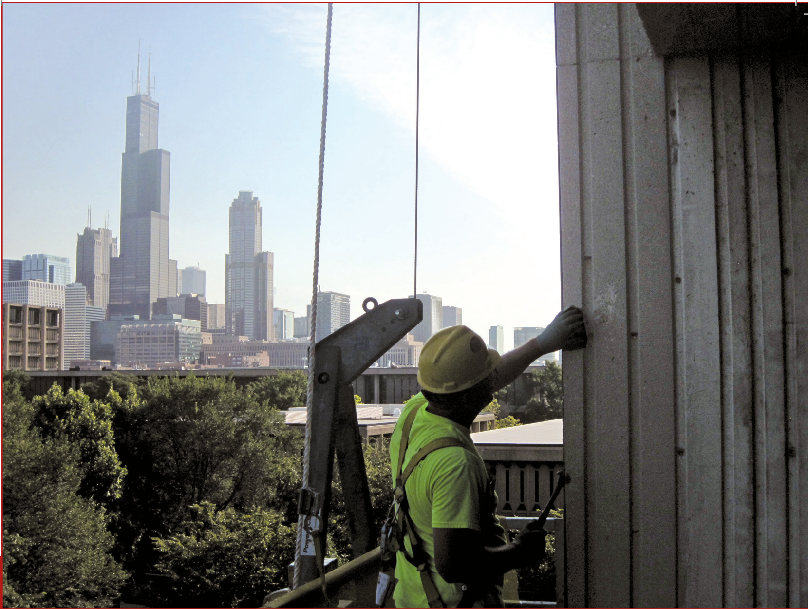
Figure 6 – Façade inspection of exposed concrete from suspended scaffold.
