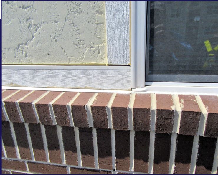
Figure 5 – These photos show window and brick veneer damages caused by wood shrinkage.
