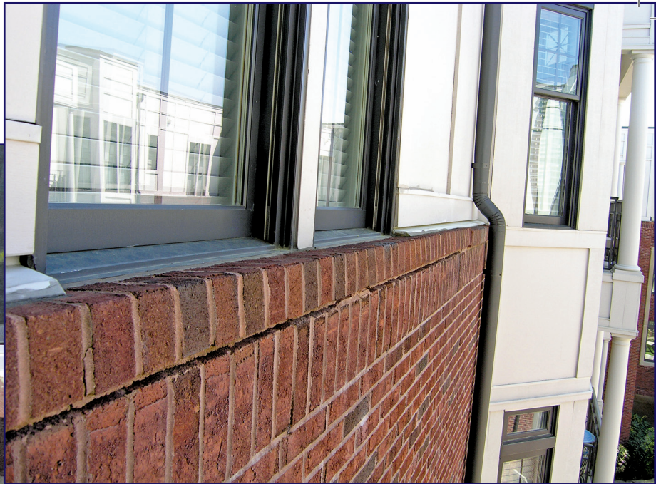
Figure 5 – These photos show window and brick veneer damages caused by wood shrinkage.
