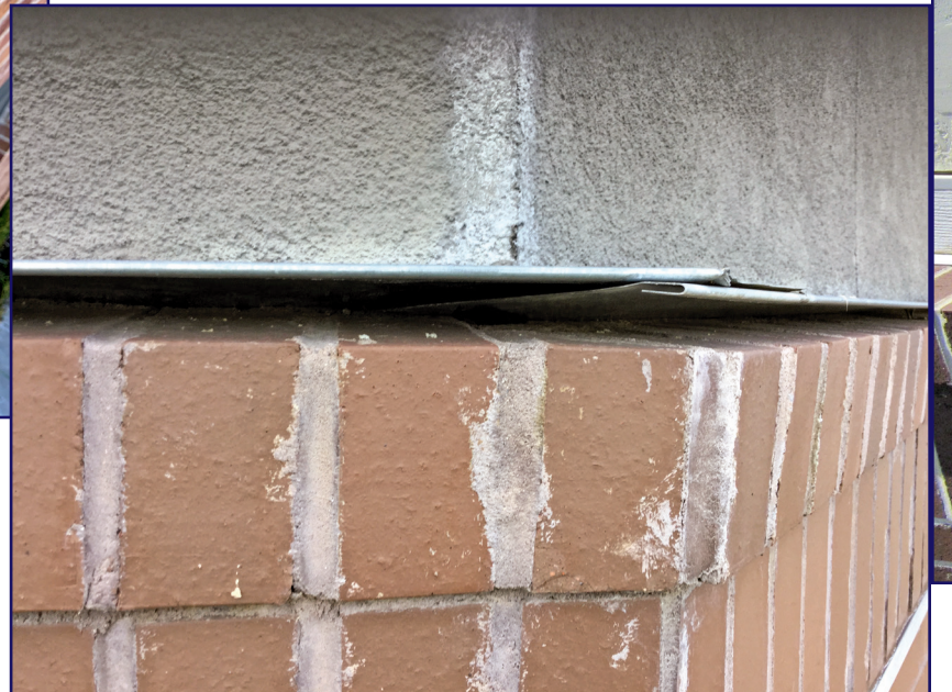
Figure 3 – These two photos show the upward rotation of flashing caused by wood frame shrinkage.
