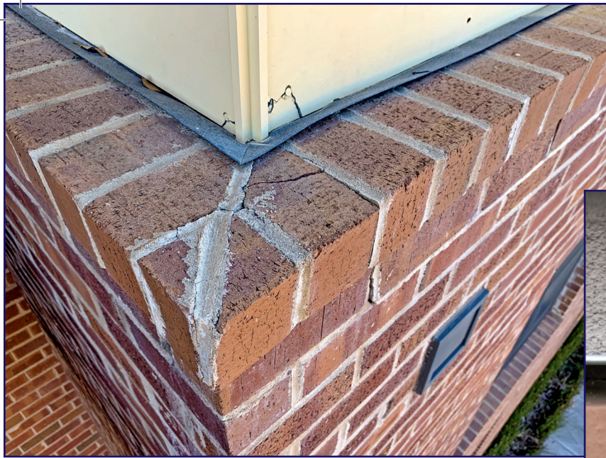
Figure 3 – These two photos show the upward rotation of flashing caused by wood frame shrinkage.
