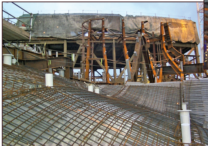
Figure 1. The structural steel framing over flexible formwork was then enveloped with shotcrete. Photo also shows a few of the many pedestals. Photo courtesy of MoPOP staff.
