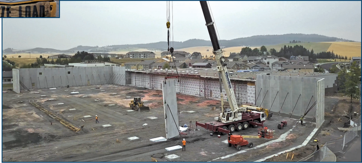
Figure 7. Composite precast concrete panel installation.
