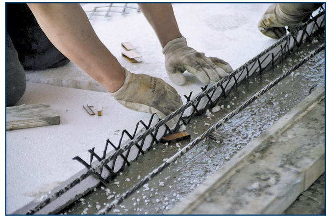
Figure 5. This close-up shows non-roughened EPS insulation and a close-up of the carbon-fiber wythe connectors.
