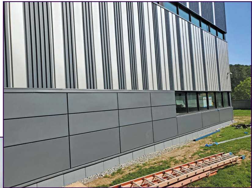
Figure 13. Completed wall depicting various metal panel types as well as insulated concrete-coated rigid insulation panels at base of wall.
