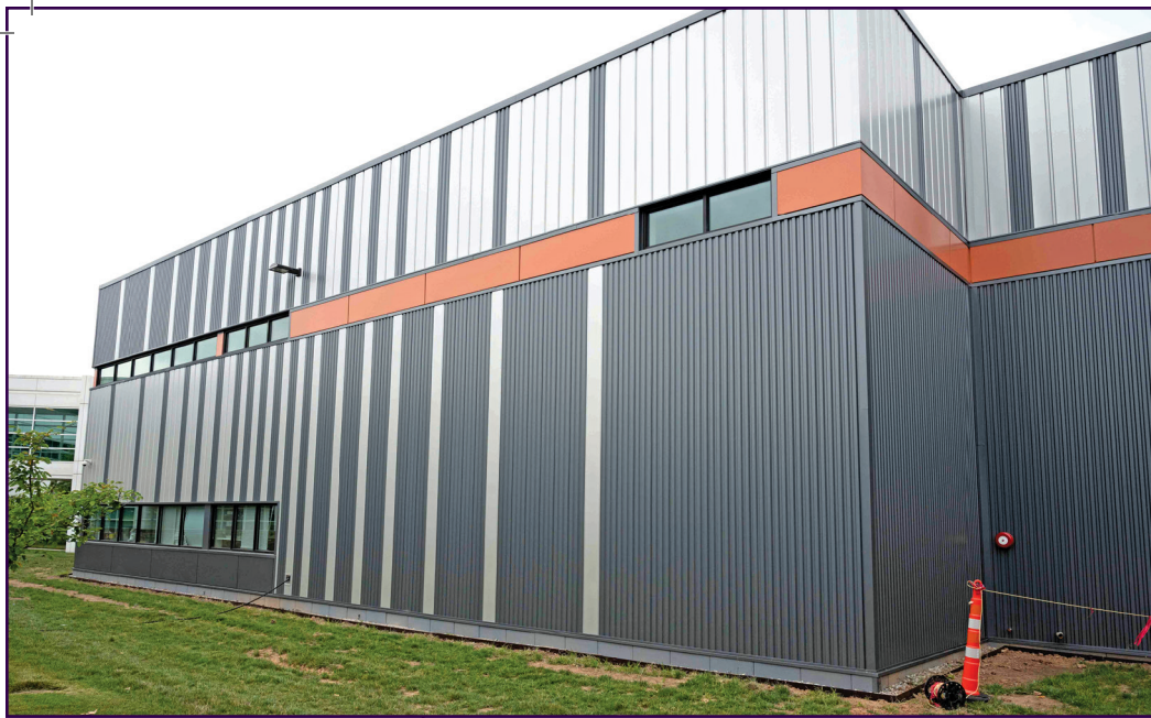
Figure 14. Completed end wall with custom colors and variation of metal building wall panels.
