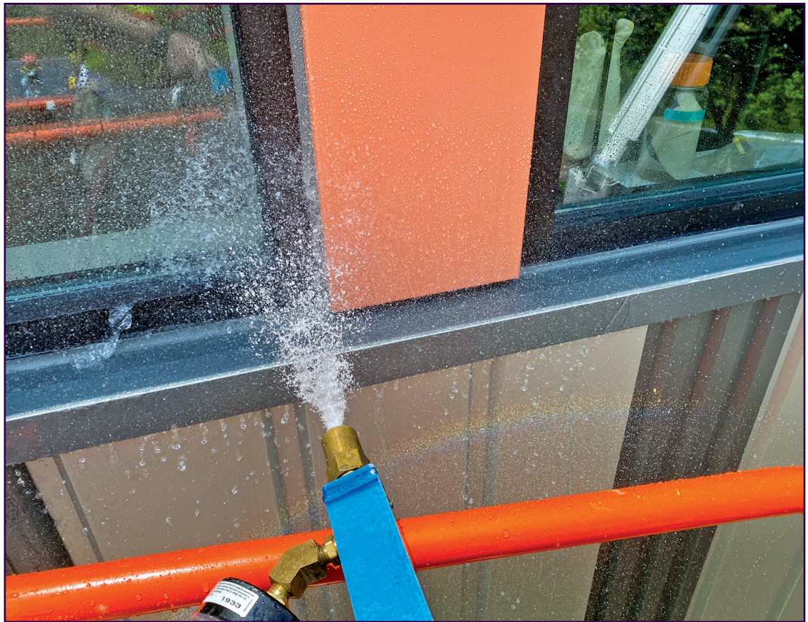
Figure 11. The installed cladding system was tested using ASTM spray nozzle techniques.
