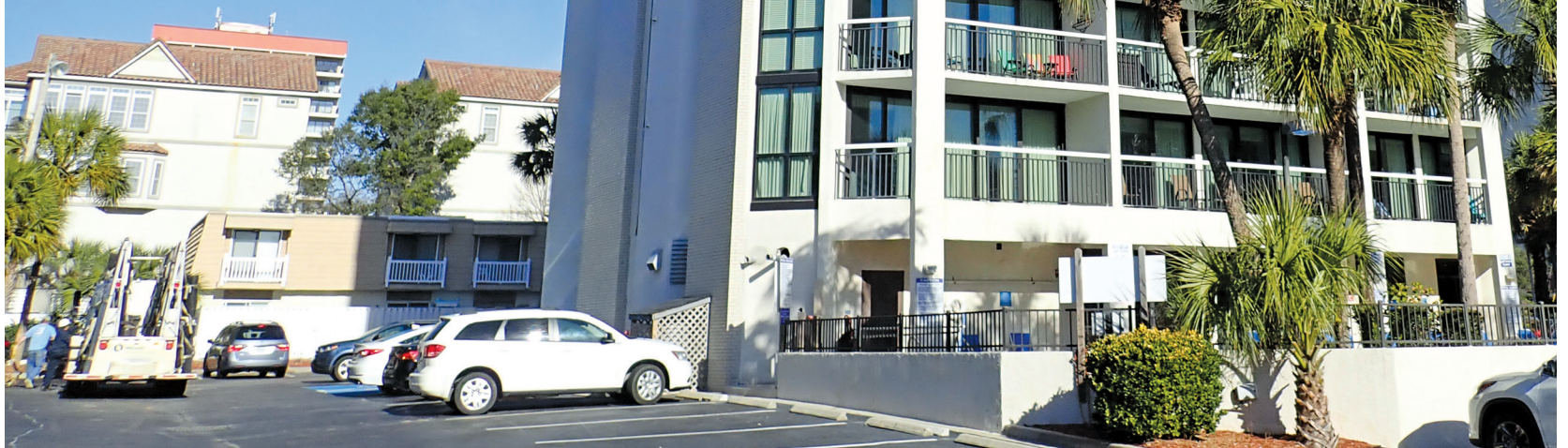
Figure 1. View of the case study building.
