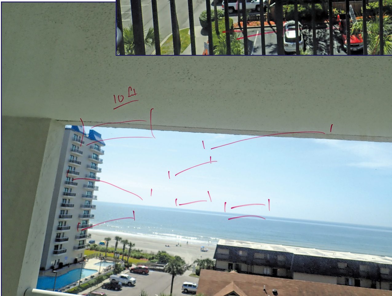
Figure 9. Views of glass surface blemishes (highlighted with red).
