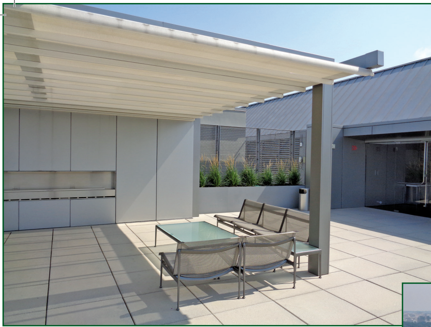
Figure 3. Existing mechanical equipment must often be relocated to make room for new amenities at existing rooftop spaces. Screen walls and planters can be used to hide or restrict access to mechanical areas. Fireplaces and other utilities will require new penetrations through the roof assembly.
