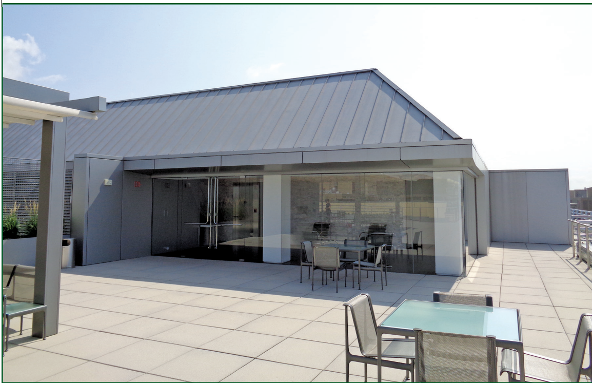
Figure 7. New interior conditioned spaces must be properly integrated into the existing primary building enclosure.
