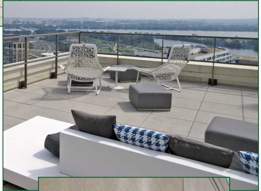
Figure 4. Consideration should be given to existing parapet heights and code requirements for guardrails. Existing parapets or guardrails may require modification to meet code requirements.
