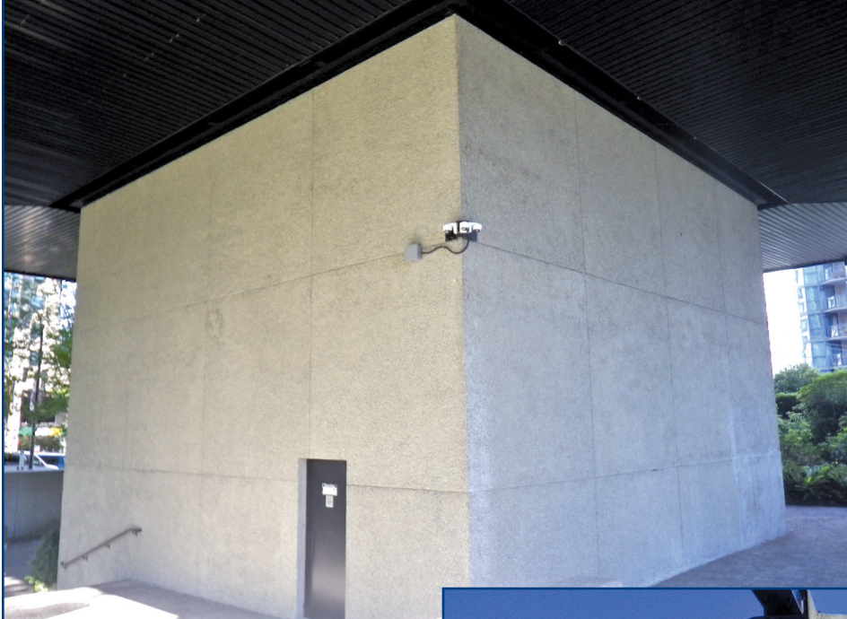
Figure 3. Central concrete core at grade.
