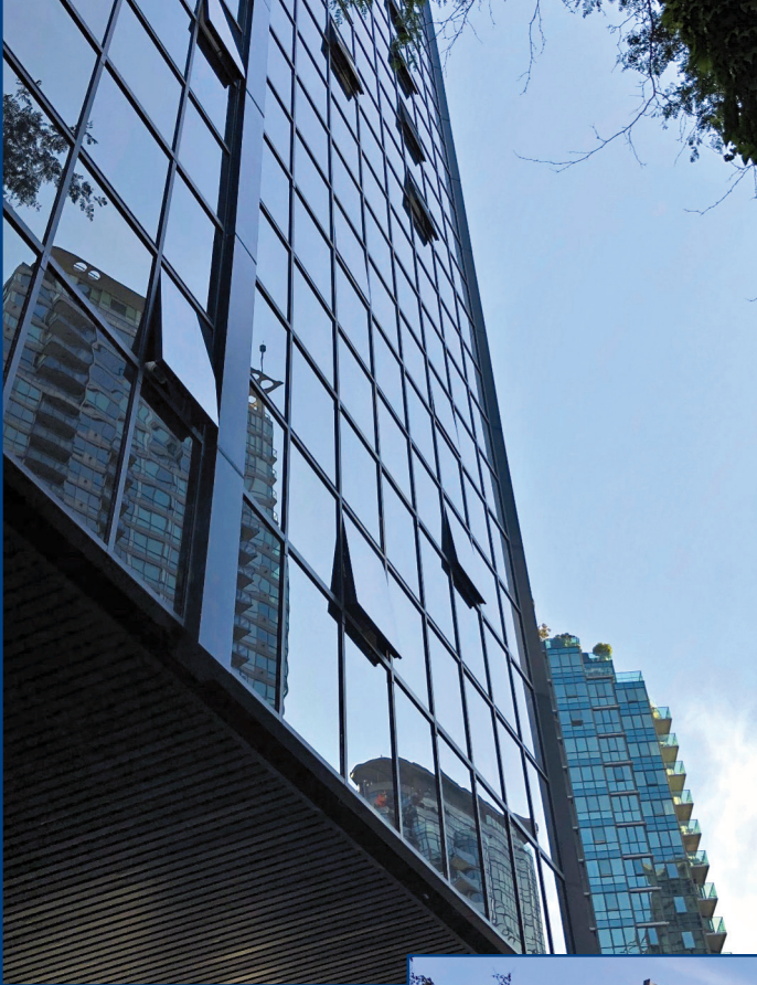
Figure 8. Cladding covers were repositioned, and custom-colored sealant strips were renewed.
