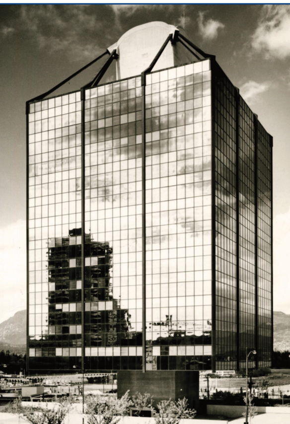
Figure 1. Westcoast Transmission Building circa 1970. Photograph courtesy of UBC Library—Rare Collections.
