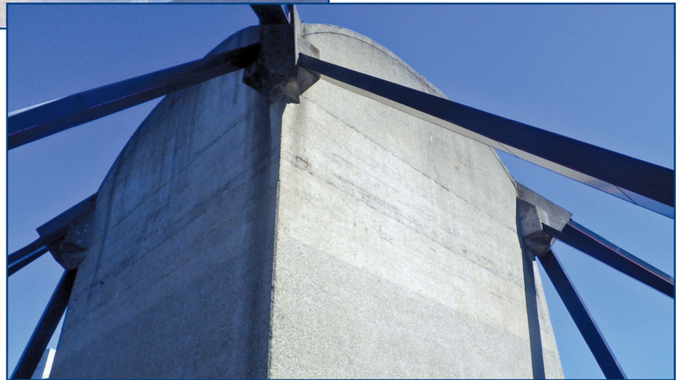
Figure 4. Exposed-aggregate concrete core at roof level.
