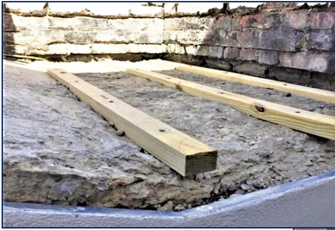
Figure 11. Proper anchoring of these new nailers required investigation of fastener holding capacity (withdrawal resistance).
