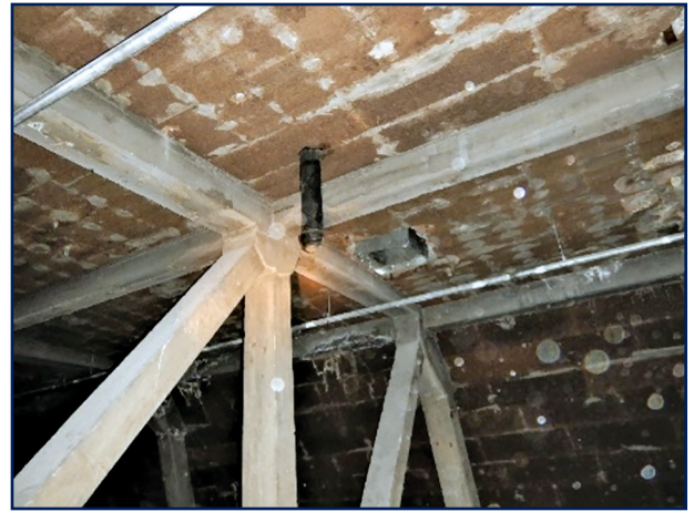
Figure 3. The underside of this deck shows the structural steel diaphragm (truss chords, web members, beams encased in concrete) on top of which the Haydite was cast, forming a monolithic arrangement and serving as a means of fireproofing. Residual cork material on the underside (described in original drawings as "insulation") was likely a bond-breaker for ease in stripping the forms.
