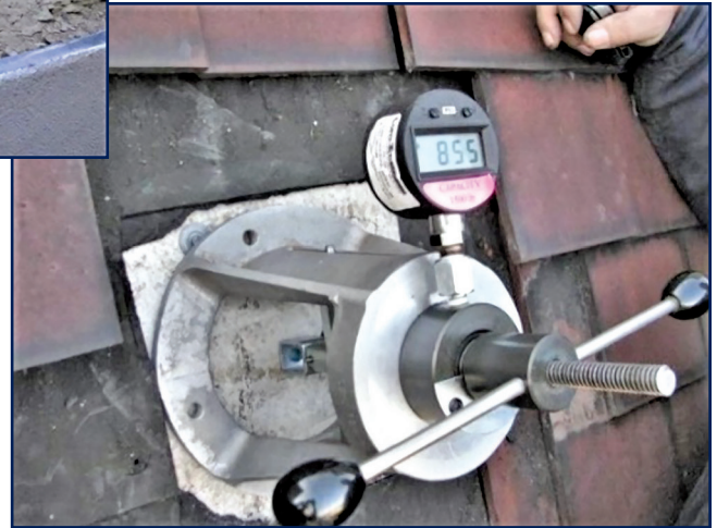
Figure 12. When in doubt, figure it out. Always deploy pull-testing to evaluate whatever fastening devices are being considered for this type of substrate.
