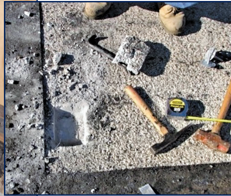
Figure 7. Something of an unusual hybrid, this 1960s-era deck is lightweight concrete over a steel formboard. While containing Haydite aggregates, this concrete is not "structural" in nature. Like more modern lightweight insulating concrete, its load-carrying capacity is mostly from the metal form-deck used.
