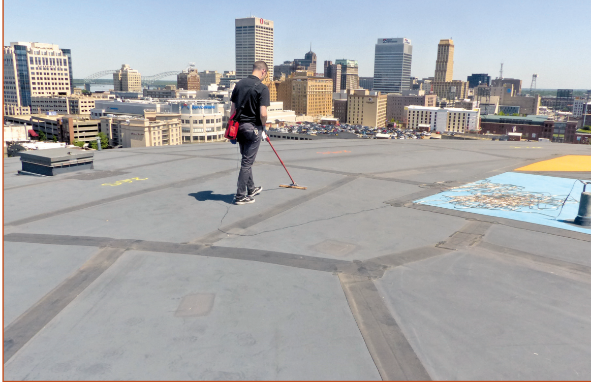
Figure 6. High-voltage electronic leak detection testing being performed.
