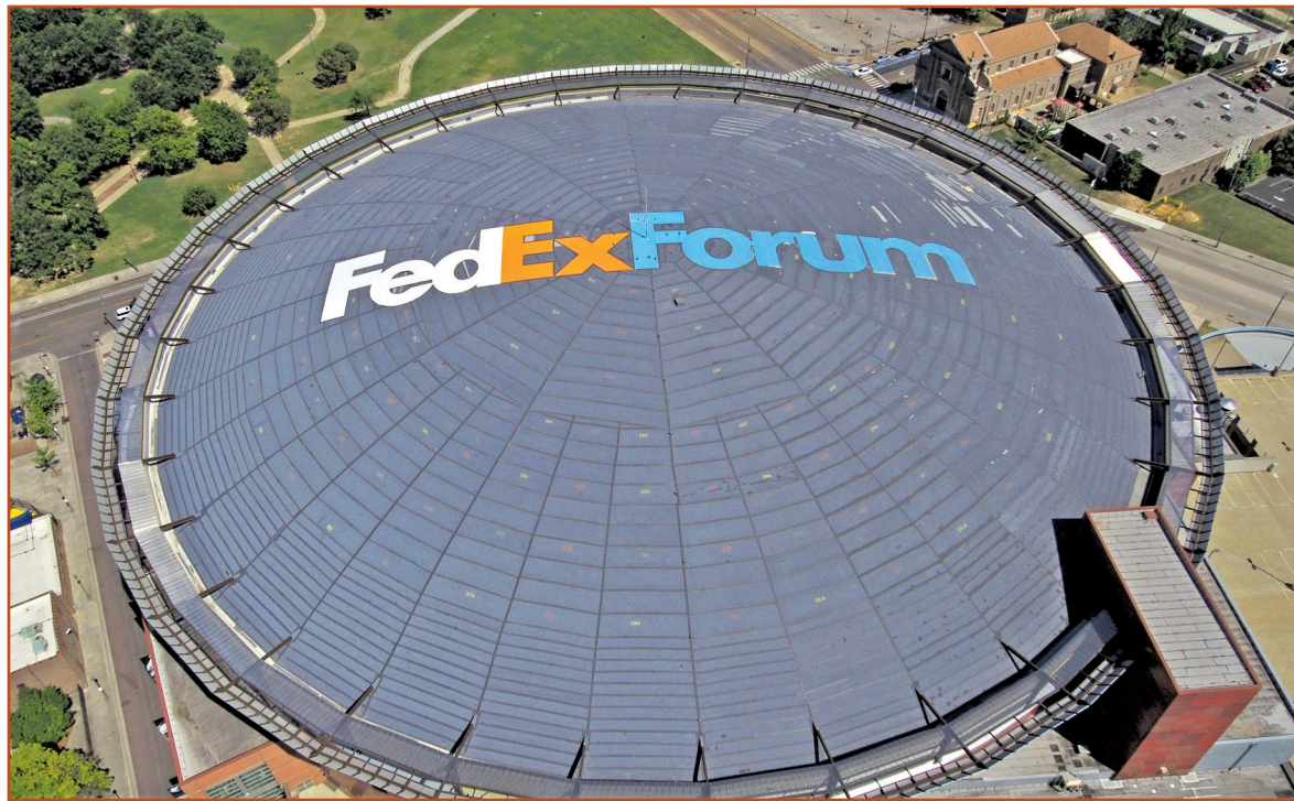
Figure 2. Overall aerial image of existing dome roof showing the roof sections.
