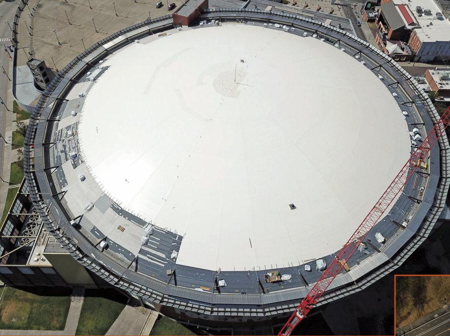
Figure 12. Work progress around the dome.
