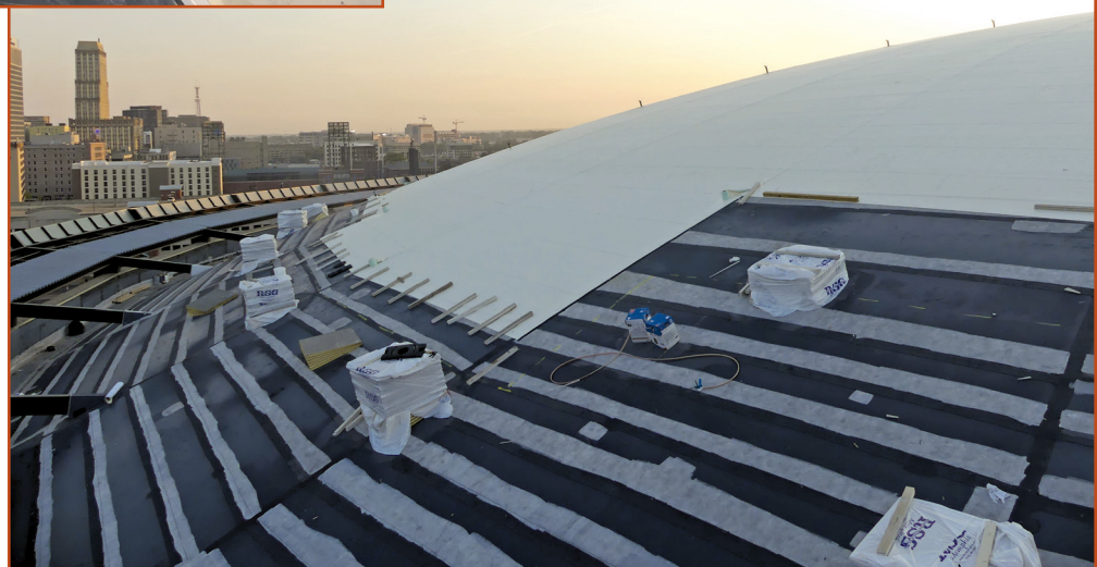
Figure 10. Roof re-cover in progress at the upper dome.
