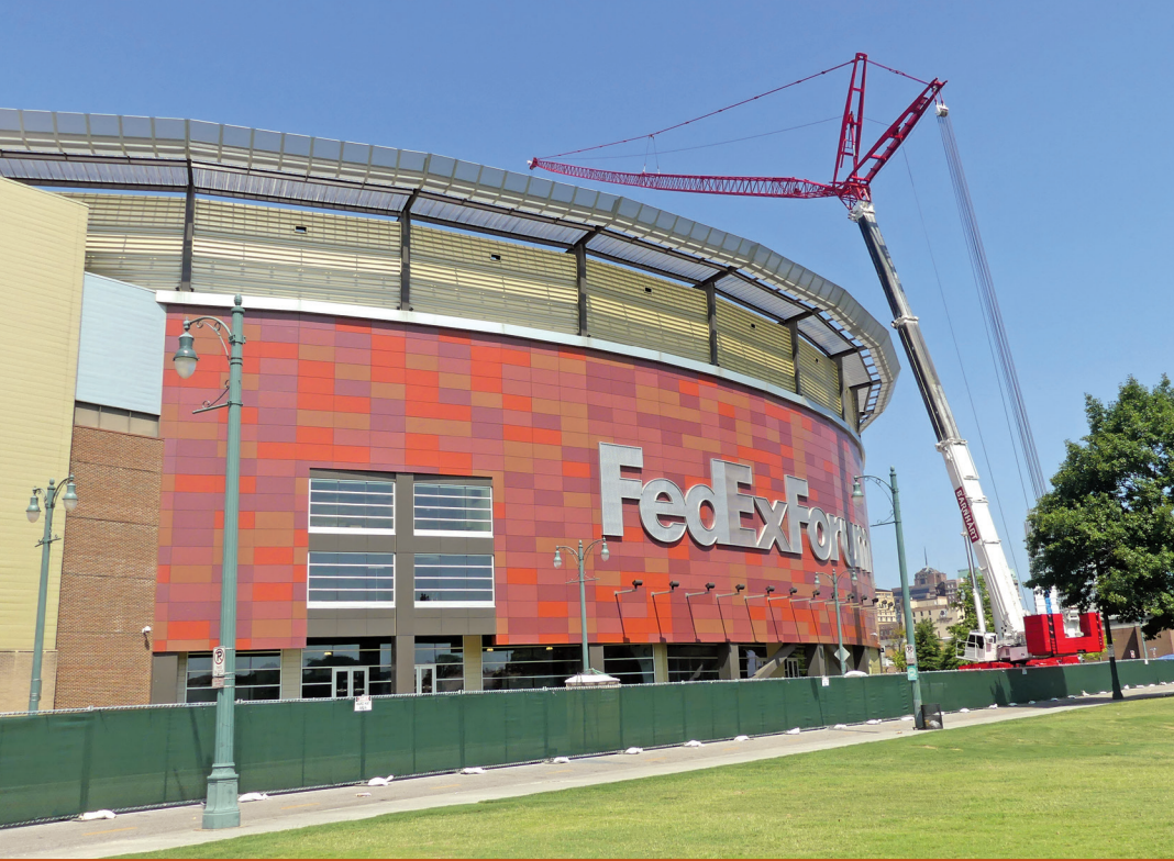
Figure 8. Staging area and crane in use.
