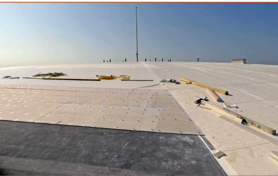
Figure 9. Roof re-cover in progress at the upper dome.
