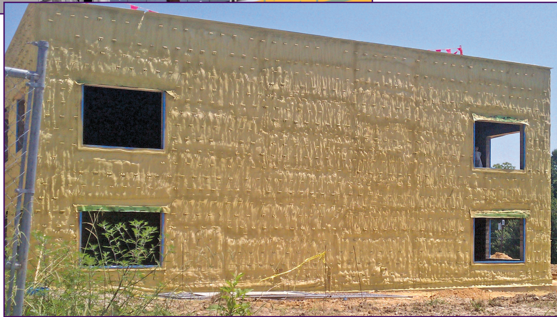
Figure 7. Spray foam air barrier.
