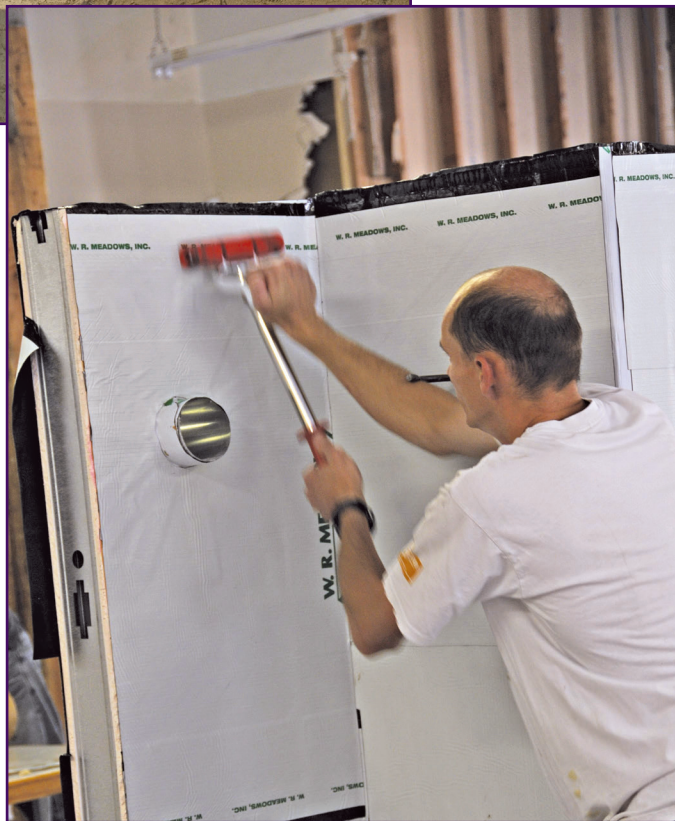
Figure 5. Self-adhered air barrier.
