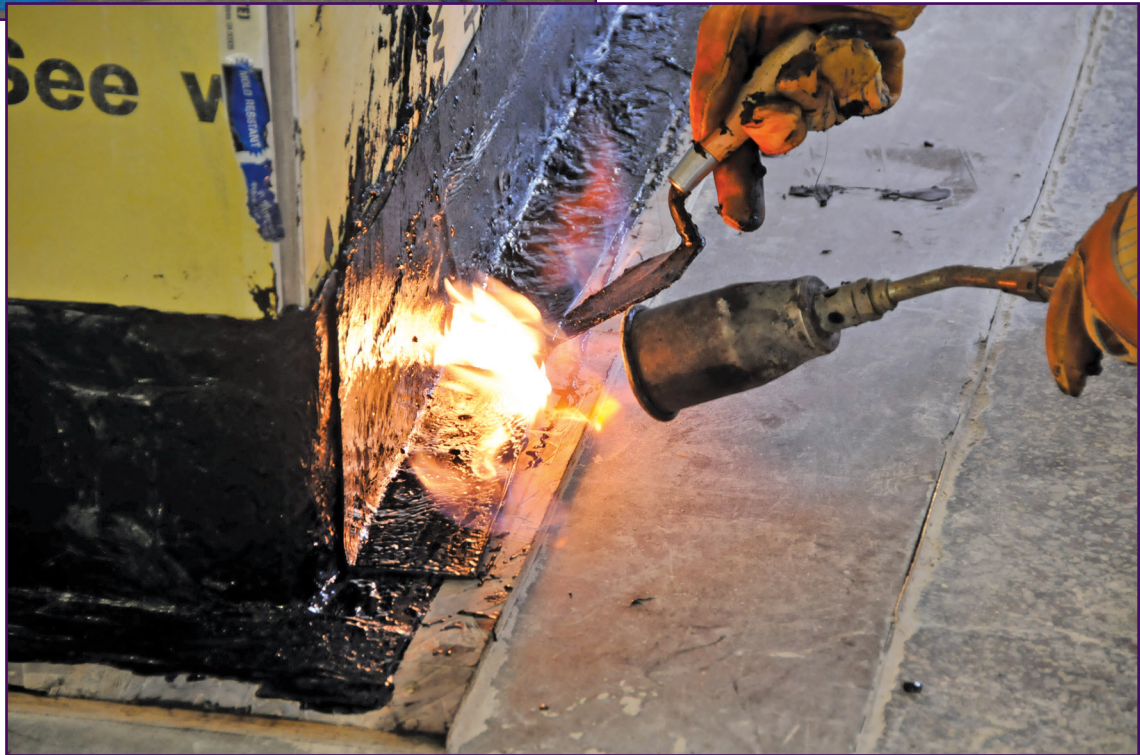
Figure 3. Torch-applied air barrier.
