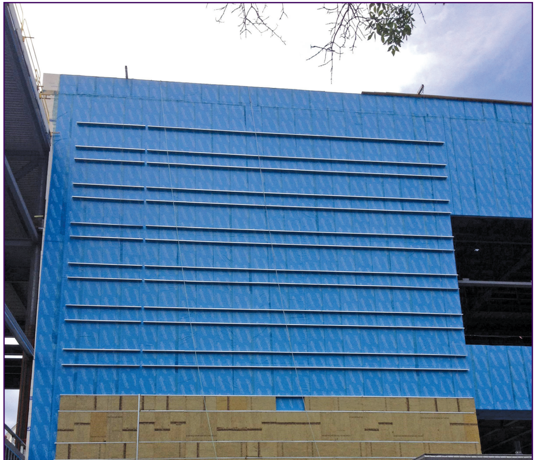
Figure 1. Installed air barrier.
