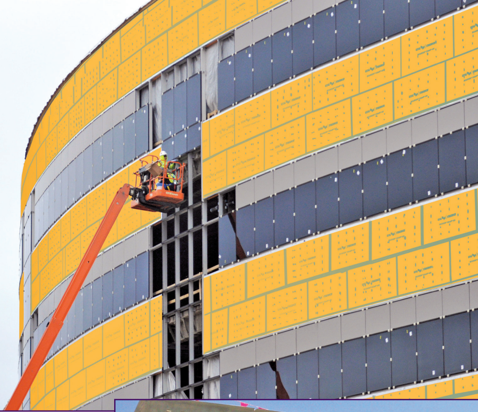
Figure 6. Gypsum board stock air barrier.
