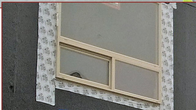
Figure 3. This photo shows an example of a nail flange window where the fluid applied is qualified as flashing and has been continued into the rough opening.
