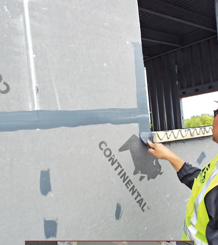
Figure 2. An accessory used to transition between joints of adjacent pieces of sheathing is visible in this photo.
