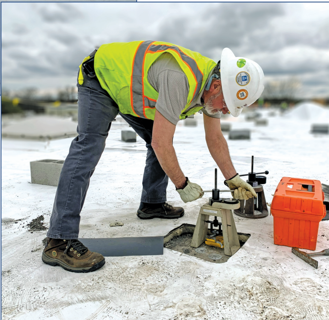
Figure 2. Pull testing to evaluate existing roof deck.
