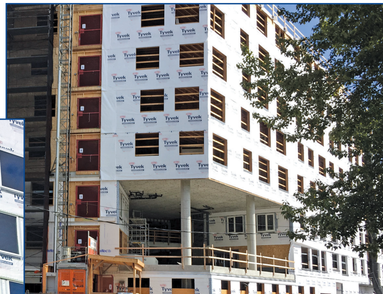
Figure 4. Mercy Housing's Mt. Baker Family Housing in Seattle, Wash., with a mechanically attached weather-resistive barrier.
