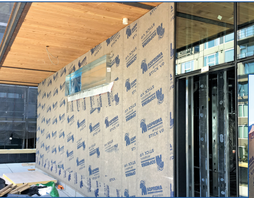
Figure 6. Ainsworth & Dunn Building in Seattle, Wash., with a self-adhered weather-resistant barrier.
