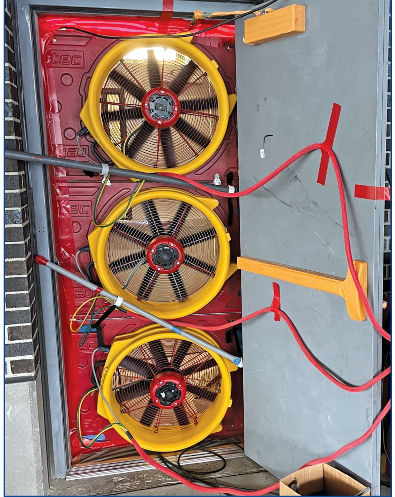
Figure 3. A typical blower door setup for the code-required whole-building air-leakage test, which is usually performed a few weeks prior to building turnover on most Walsh Construction Co. projects.
