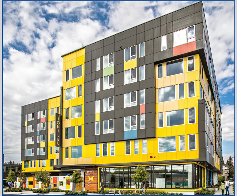
A typical Walsh Construction Co. project, the Low Income Housing Institute's Tony Lee Apartments—Lake City Family Housing in Seattle, Wash., includes five stories of wood framing over a post-tensioned concrete deck.
