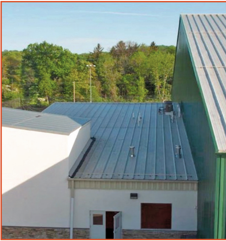
Figure 4. While roof loads are usually less than ground loads, aerodynamic shade (drift load, shadow load) can cause roof design loads on a lower roof to be several times greater than that of ground snow.
