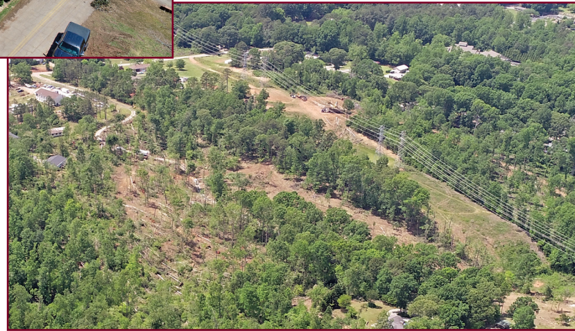
Figure 13. Damage adjacent to residence R-2.
