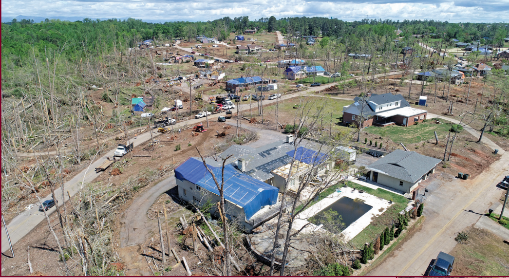
Figure 12. Damage adjacent to residence R-1.
