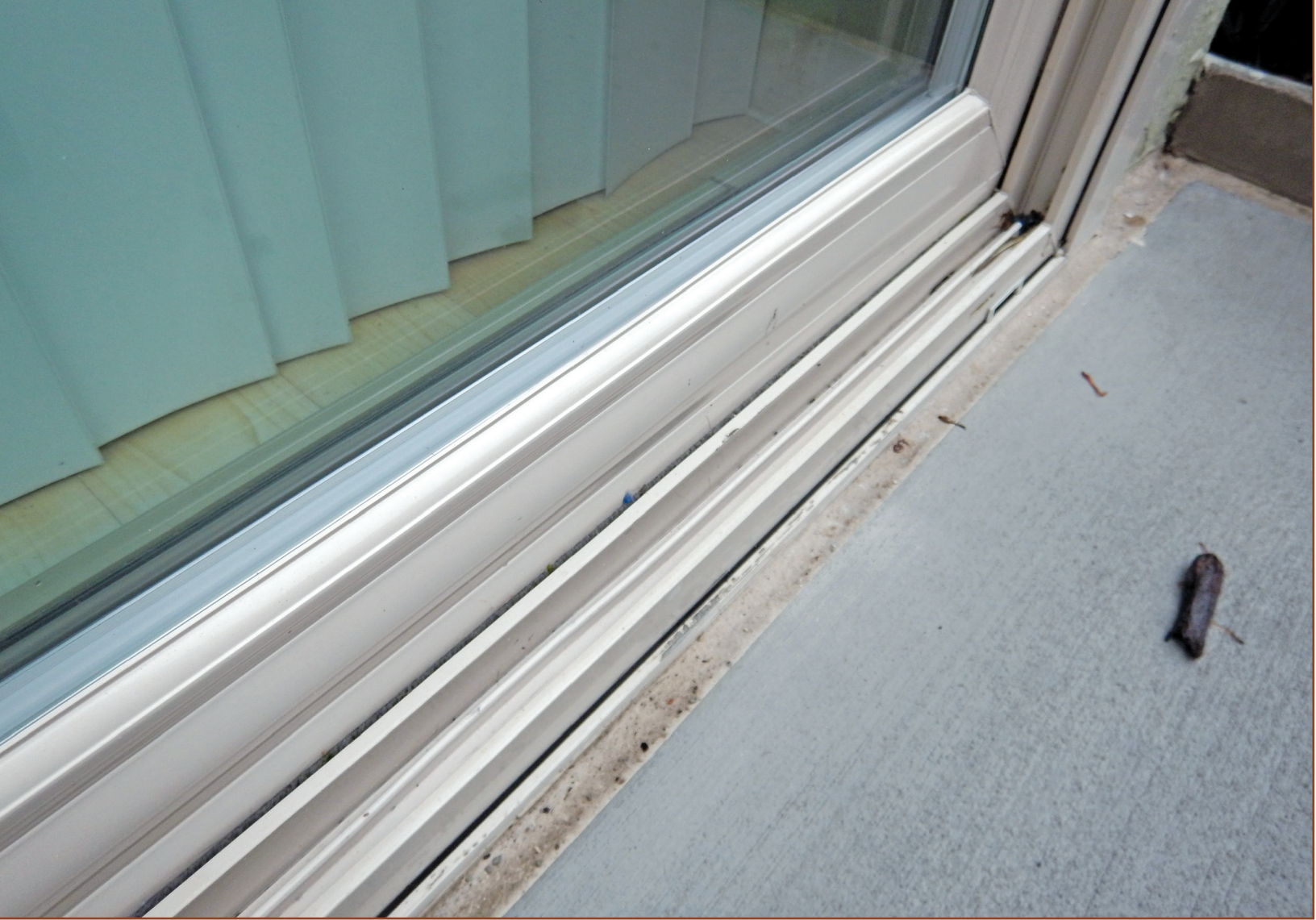
Figure 10. Sliding door's doorframe at the sill.
