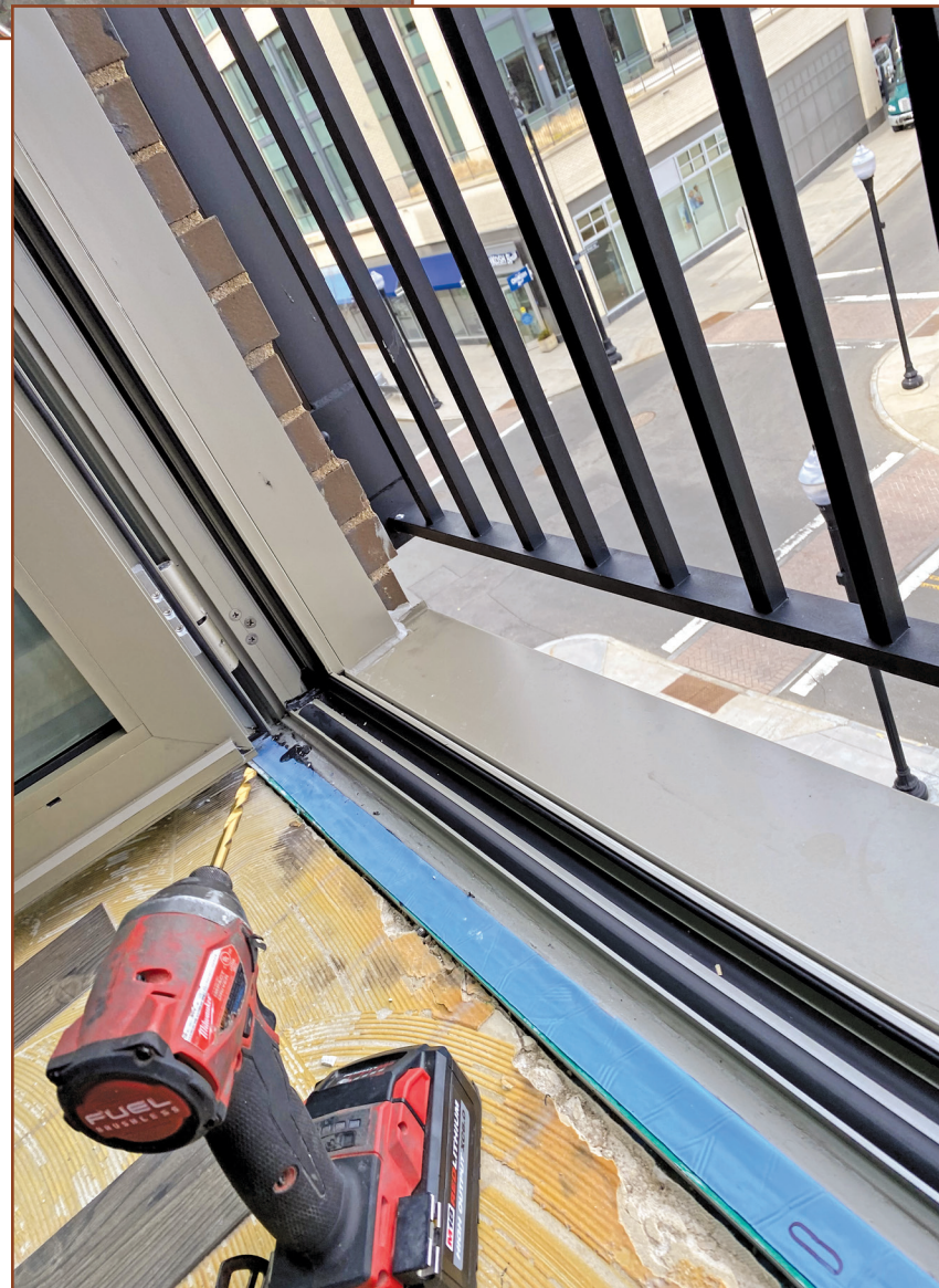
Figure 9. Door sill-to-jamb intersection of a terrace-style door installed at a Juliet balcony.
