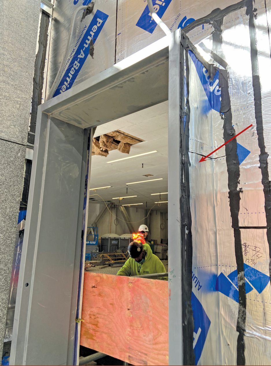
Figure 2. Metal flashing (red arrow) installed continuously around a hollow metal door's perimeter and covered with weather barrier.
