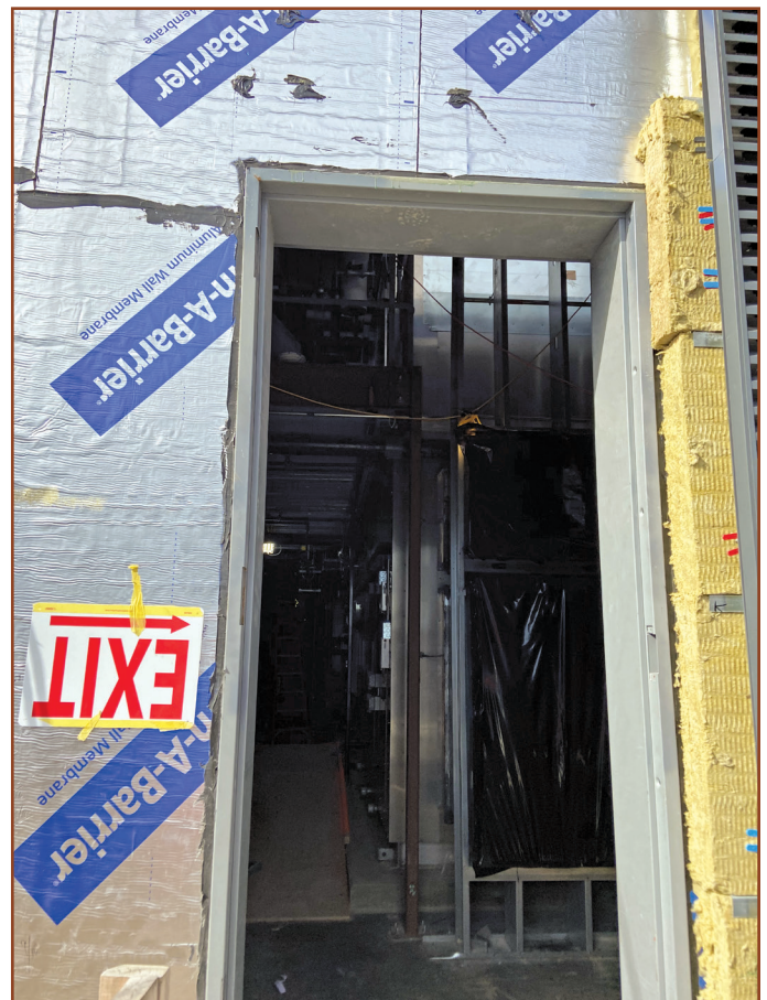
Figure 7. Hollow metal doorframe.
