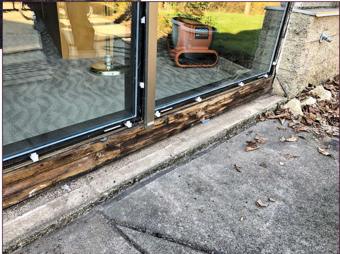
Figure 5. Because the storefront window system lacked proper sill pans and end dams, water could escape into the wall below the sill, causing damage to stacked wood framing. Photo courtesy of Inspec.
