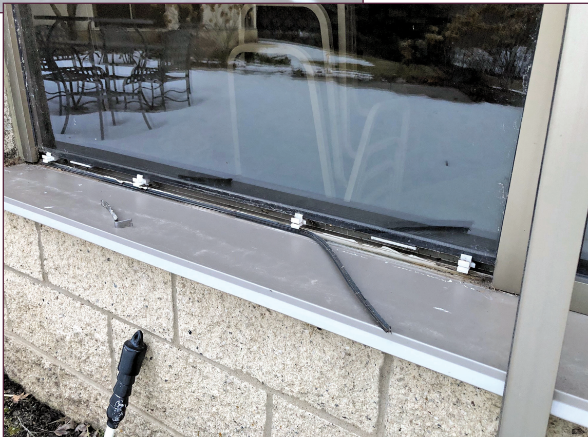
Figure 3. The window frames did not incorporate a sill pan to direct water to the exterior. The flashing shown stopped at the front of the window, where it met the gasketing and no end dams were incorporated. Note the previous attempt to seal the window system from the outside where the flashing met the gasketing. Photo courtesy of Inspec.
