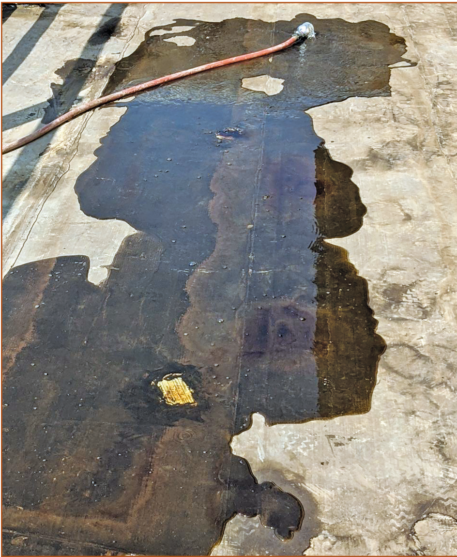
Figure 5. Flood testing with a soaker attachment.
