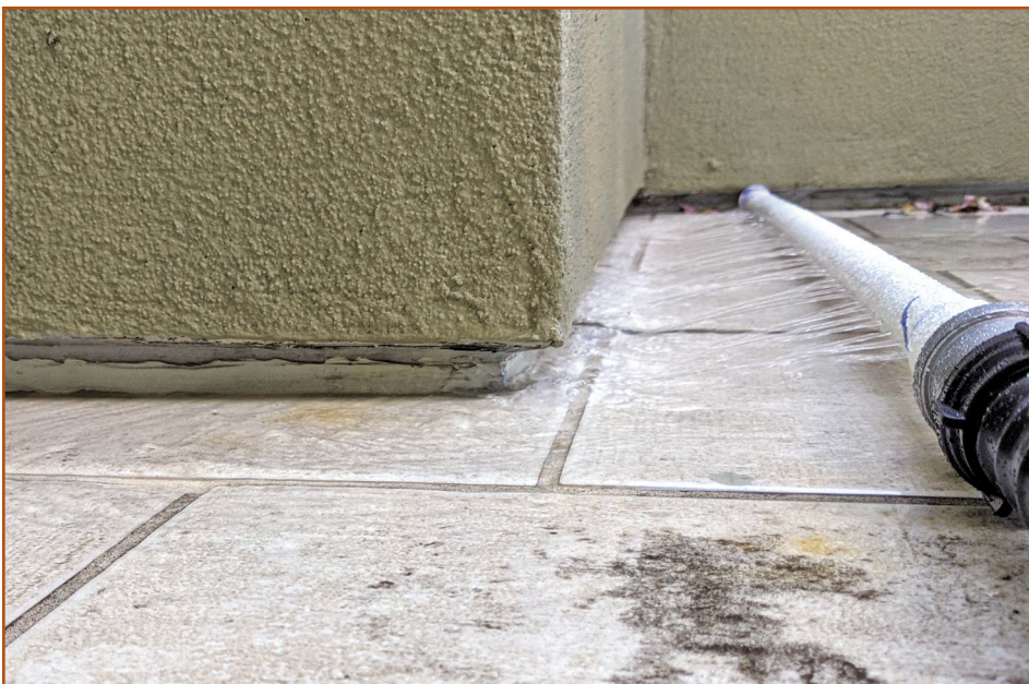
Figure 3. Testing a deck-to-wall transition using an ASTM E514 wand.
