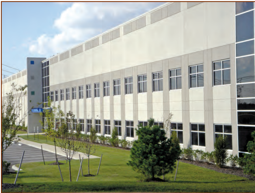
Figure 6. Example of a project produced by precaster with category AD certification from the Precast/Prestressed Concrete Institute Architectural Certification Program—Middlesex Center Warehouse in Jamesburg, New Jersey. Photo courtesy of Altus Group and Oldcastle Precast.
