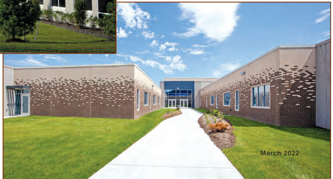
Figure 7. Example of a project that would be best produced by precasters with category AC certification from the Precast/Prestressed Concrete Institute Architectural Certification Program—DC West Elementary School in Valley, Nebraska. Photo courtesy of Jacia Phillips | Arch Photo KC and Enterprise Precast Concrete.
