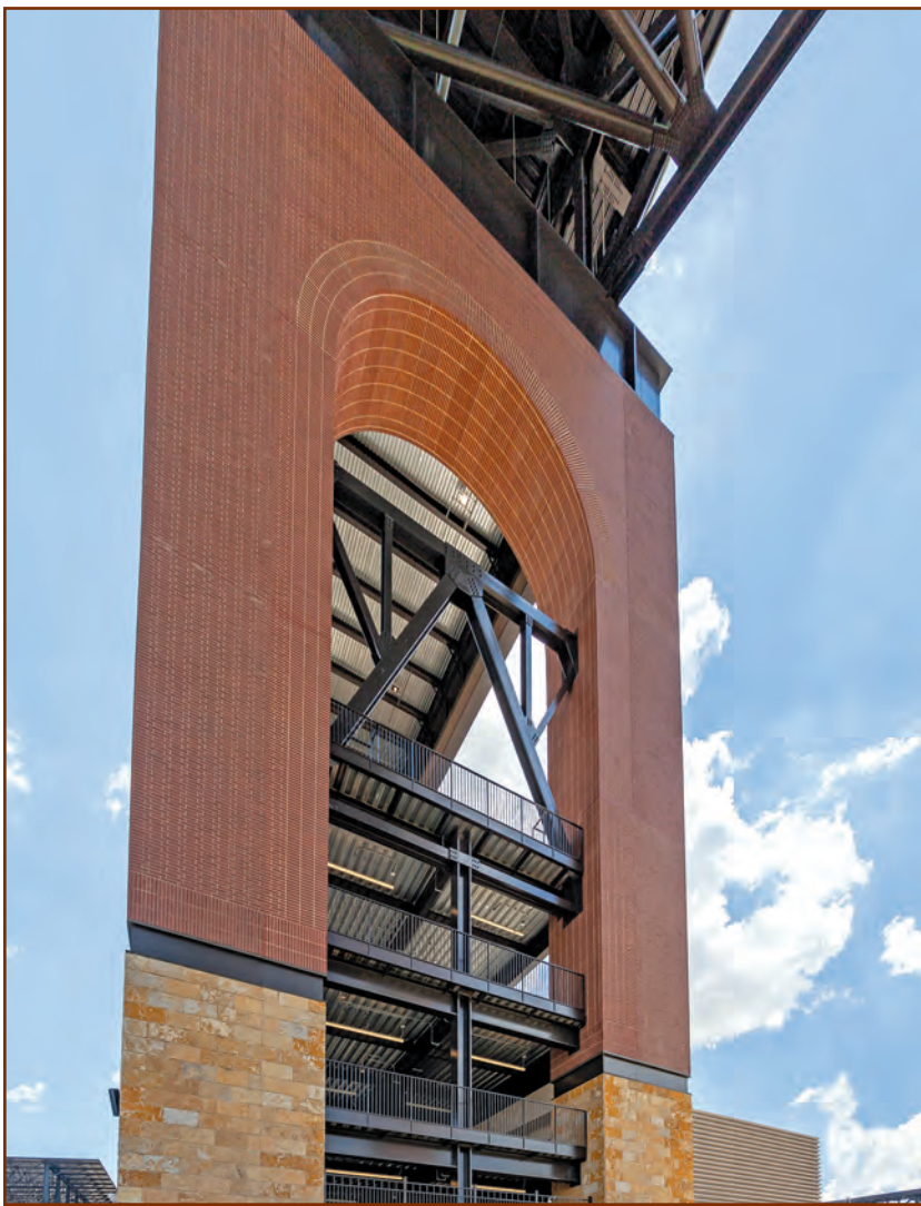
Figure 2. Examples of thin brick formliners and applications used at Globe Life Field ballpark, home of the Texas Rangers, in Arlington, Texas. Photo courtesy of Jacia Phillips | Arch Photo KC and Enterprise Precast Concrete.
