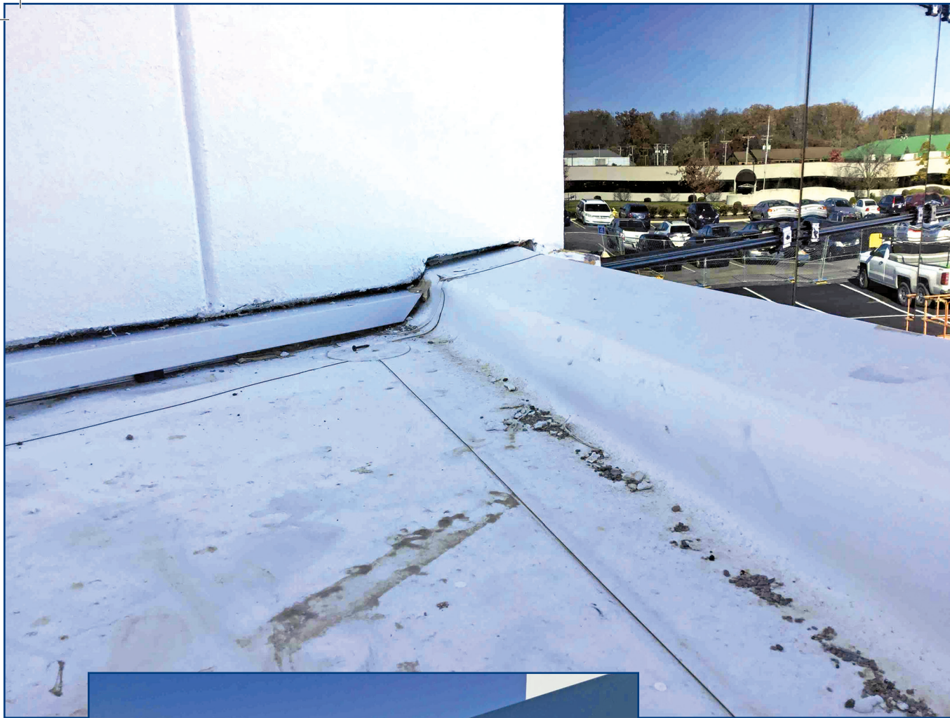
Figure 6. A thermoplastic polyolefin-clad parapet wall transition to exterior insulation and finish system condition.
