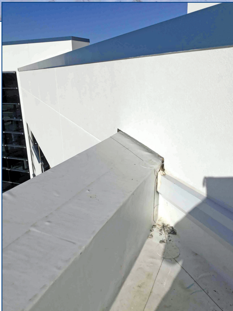
Figure 7. A thermoplastic polyolefin-clad parapet wall transition to exterior insulation and finish system condition.
