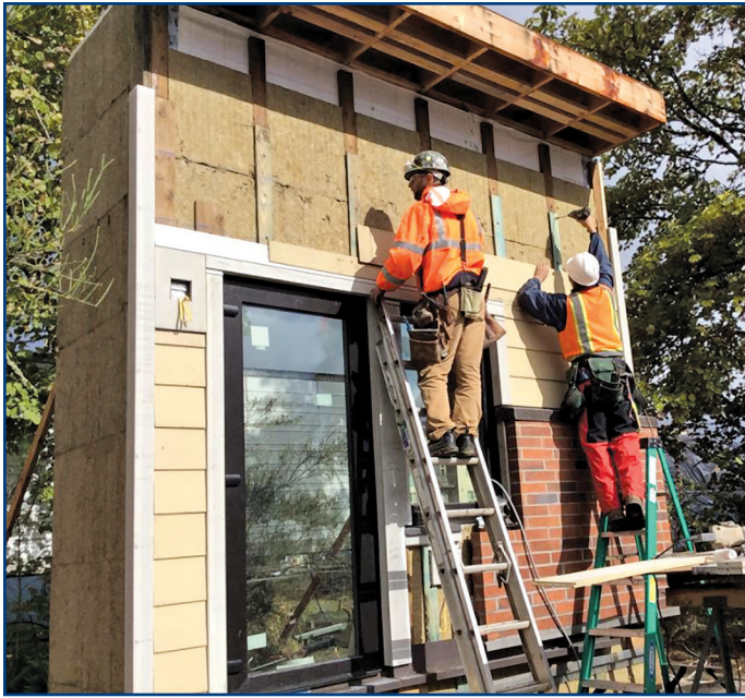
Figure 1. Mock-up panel illustrating several key attributes of a comprehensive evaluation of an exterior wall and roof assembly. Figure courtesy of Walsh Construction Co.
