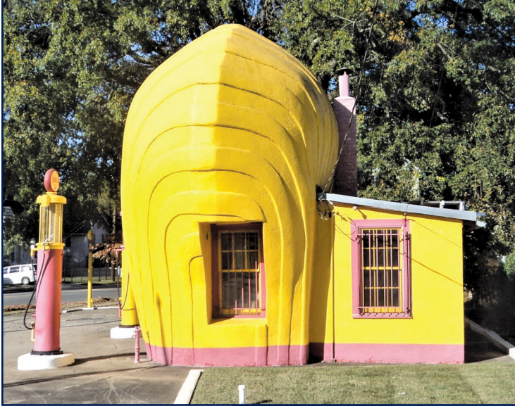
Figure 2. Two views of a uniquely structured gas station. A National Historic Landmark near Winston-Salem, North Carolina, exemplifies a shell-like design. The exterior is more of a wall than a roof, there is no membrane, and exterior weatherproofing is merely a paint coating.
