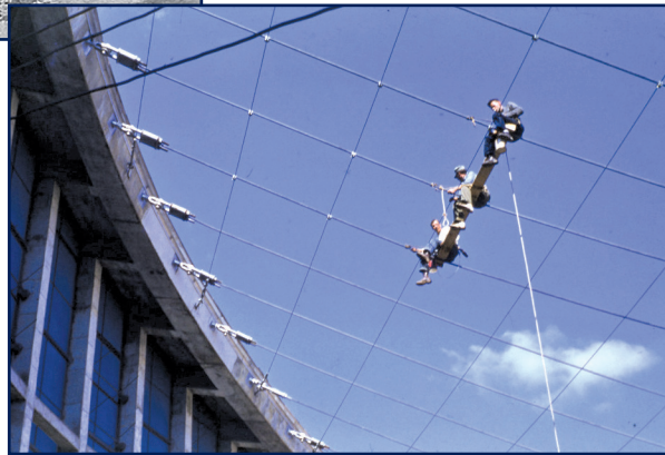
Figure 9. J. S. Dorton Arena, which was the first structure in the world to use a cable-supported roof, has an asbestos-coated steel deck that is bolt-clipped onto the grid of draped steel cables. Figure: James L. Brandt Papers, MC 00472, NC State University Libraries Special Collections Research Center.
