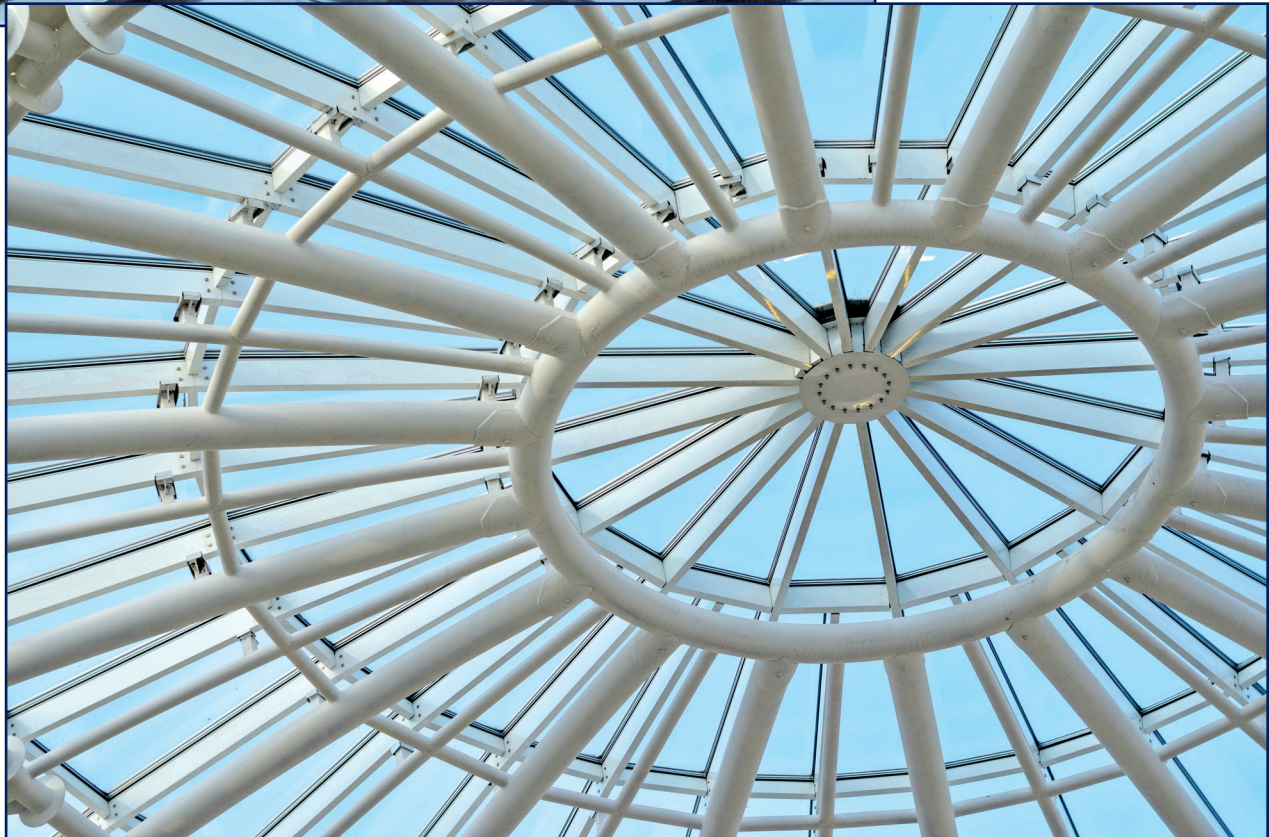
Figure 5. Under rooftop service loads, the oculus ring is in compression. Further down the slope, ribs transfer load to the perimeter ring, which experiences tension.
