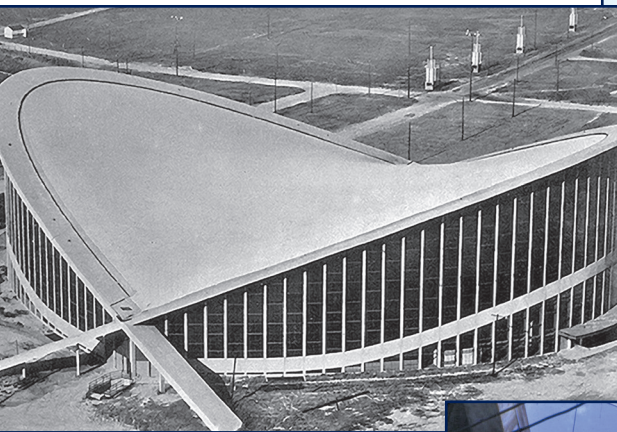
Figure 8. Completed in 1952, the J. S. Dorton Arena in Raleigh, North Carolina, is a notable hyperbolic paraboloid. The convergence of the two concrete parabolas creates a challenge for the management of stormwater runoff. Figure: https://ncmodernist.org/nowicki.htm .
