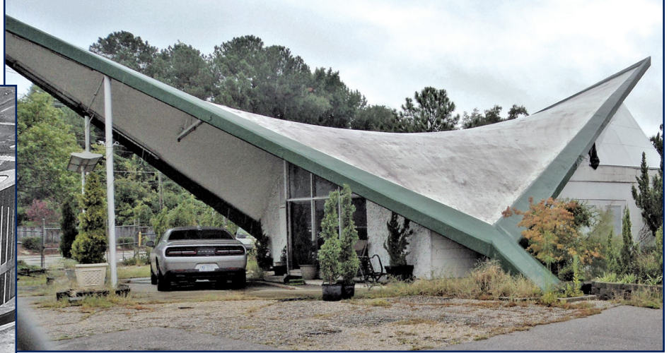
Figure 10. Paraboloids are often constructed from cast-in-place concrete with only a coating applied. Because of the generous slope across the entire shape, coating can perform satisfactorily if a quality product is selected and applied well. However, it is critical to correctly size the internal drainage devices to manage stormwater.
