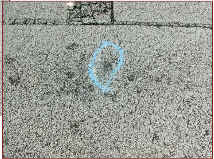
Figure 31. A closer view of the hail-caused granule loss on the same project as Fig. 30.
