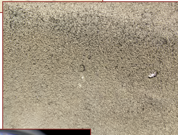
Figure 37. A closer view of localized granule loss occurring as a result of contaminants from bird droppings.
