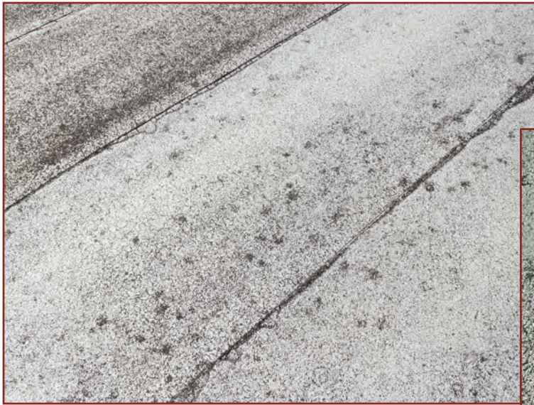
Figure 30. An example of localized granule loss on an aged modified bitumen roof.
