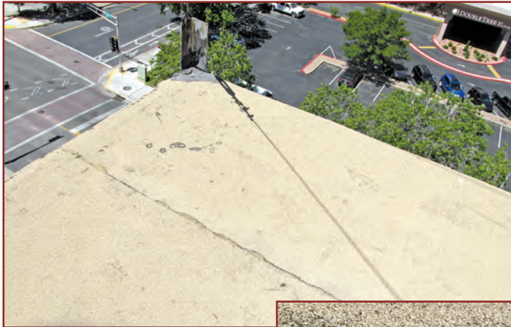
Figure 36. Localized areas of granule loss tend to be in specific areas where birds congregate.
