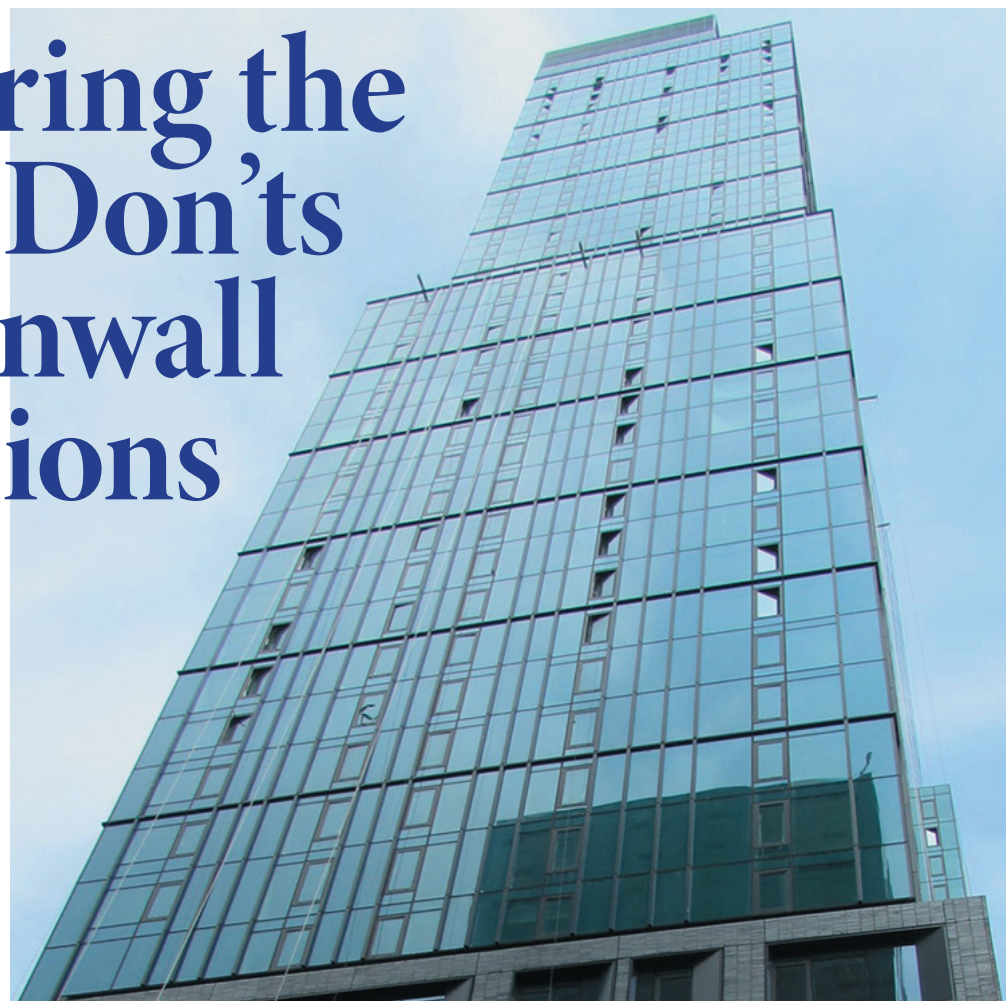
Figure 1. Unitized curtainwall enclosure.
