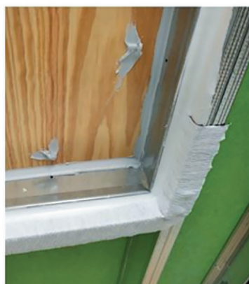
Figure 8. Mock-up 6, round 1 testing, mechanically fastened WRB system. Note: WRB = water-resistive barrier.
