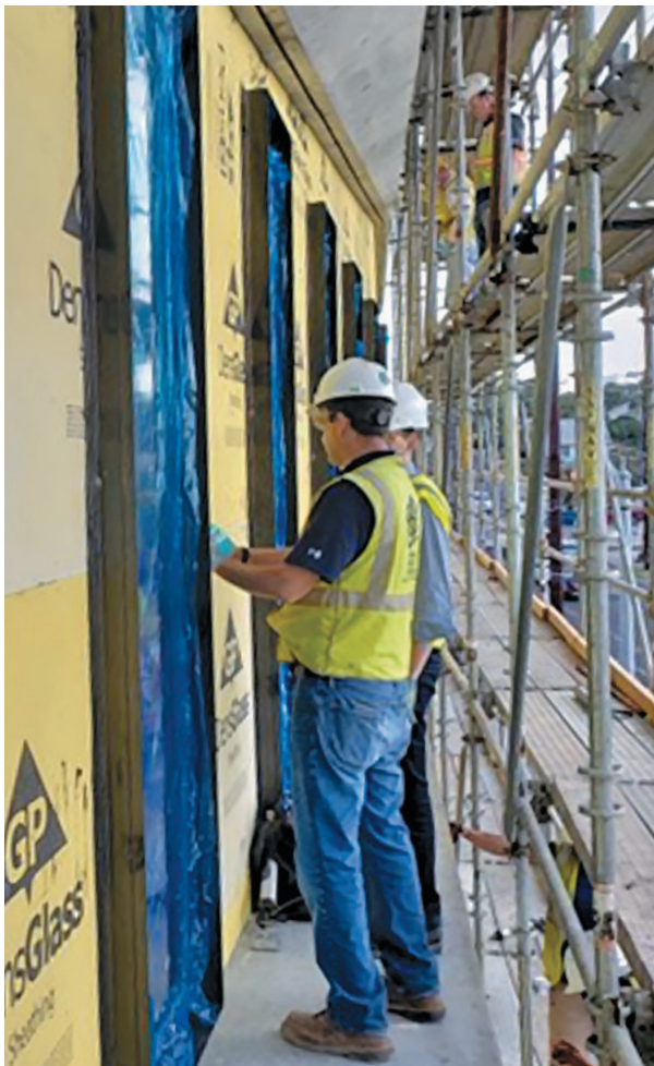
Figure 13. Commercial flanged window installation.
