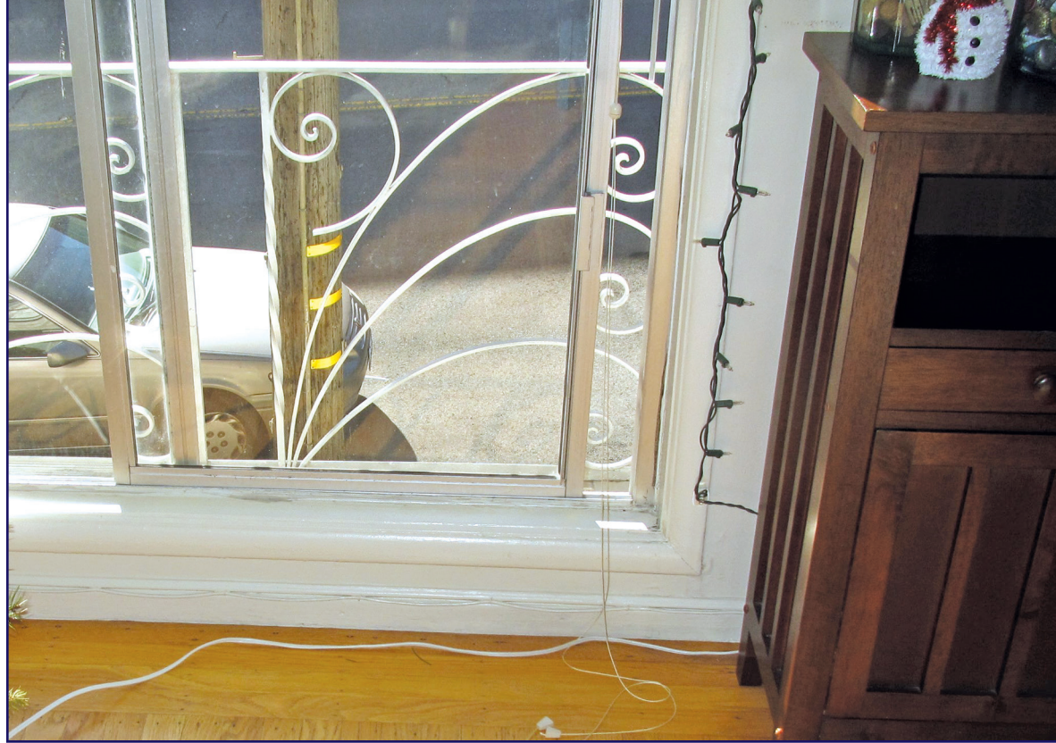
Figure 9. The invitingly low (7 in.) interior threshold height for the operable sashes at these circa-1972 horizontal sliding aluminum windows encouraged tenant access to the two balconies. Note: 1 in. = 25.4 mm.
