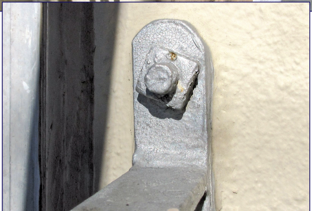
Figure 6. This hanger screw at the opposite end of the lower balcony from the screw in Fig. 5 did not exhibit evidence of axial (overturning) overloading and withdrawal comparable to that shown in Fig. 5.
