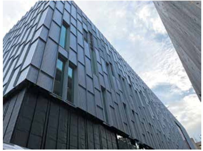
Figure 10. Open-joint cladding and furring spaced to accommodate drift. Figure 11. Panelized wall facade nearing completion.
