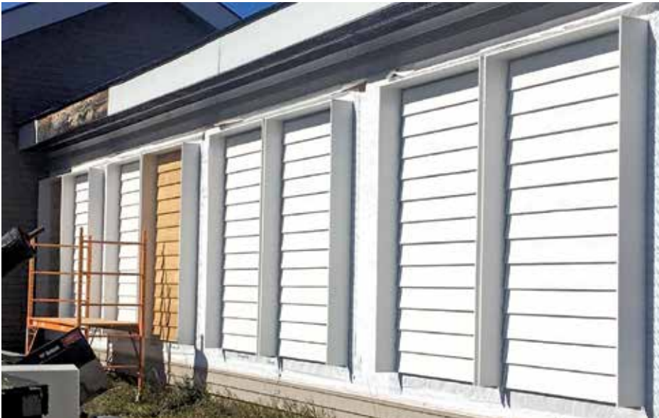
Figure 3. Exterior view of baseline walls depicting cedar siding before wall retrofits.
