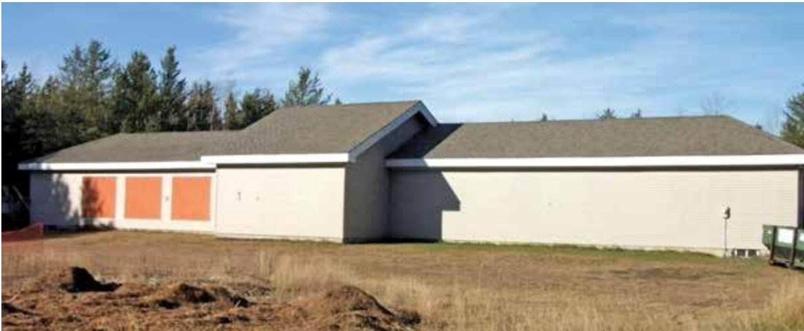
Figure 1. The Cloquet Residential Research Facility was used for the in situ testing of retrofit wall assemblies.
