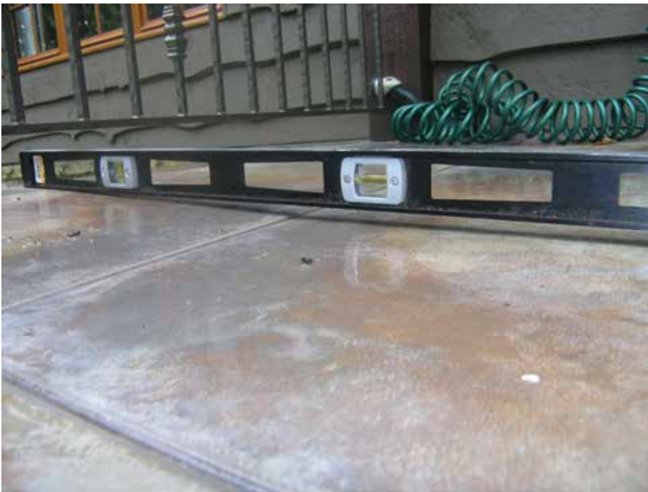
Figure 3. Ponded water at a balcony edge.
