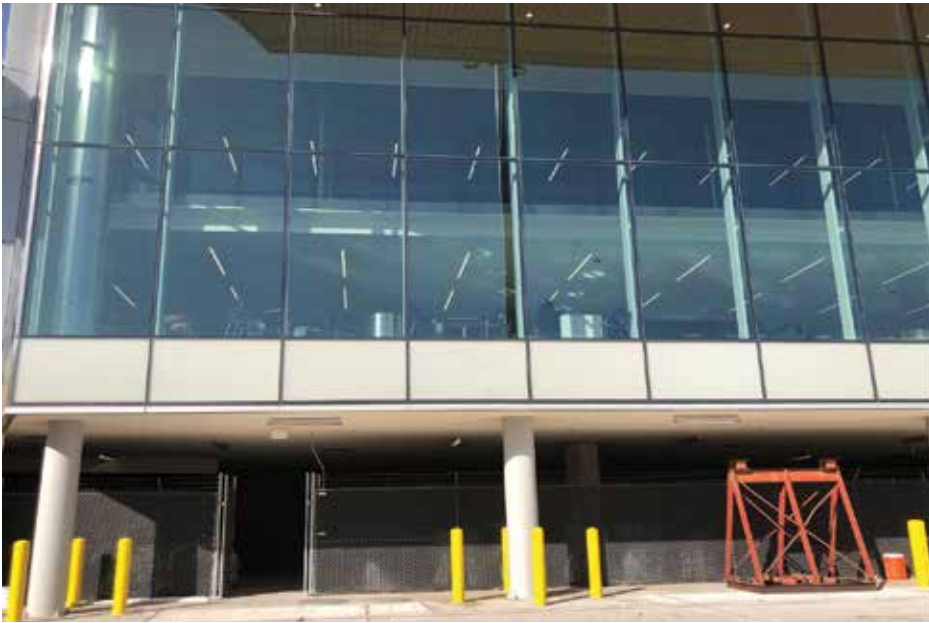
Figure 2. Exterior curtainwall drops below the interior floor to heighten design.
