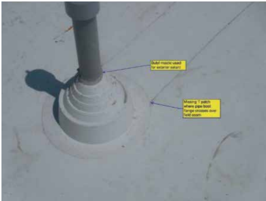
Figure 2. Example of an incorrectly installed prefabricated pipe boot penetration. The wrong sealant was used at the exposed surface against the pipe, and T patches are missing where the pipe boot flange crosses field seams.
