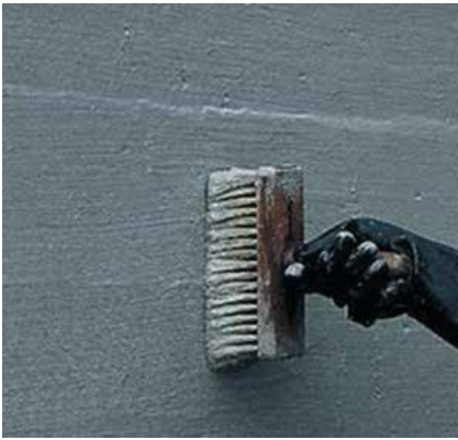
Figure 4. Crystalline waterproofing being applied by brush.
