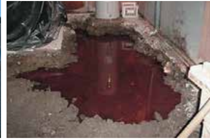
Figure 2. Oil (petroleum) infiltration can be identified by color and odor.
