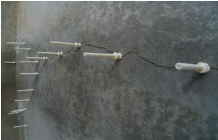
Figure 7. Port installation for epoxy injection.
