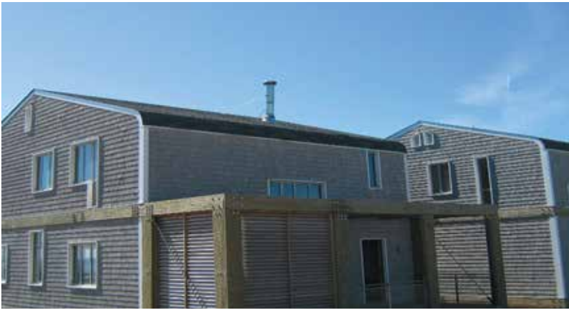
Figure 1. Absence of gutters can cause additional recharging of soil from roof runoff.
