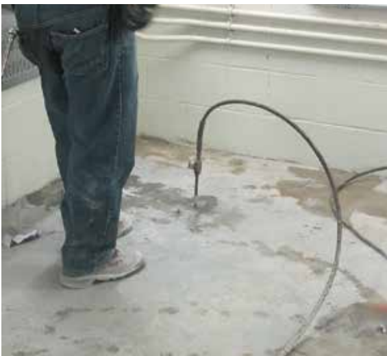
Figure 8. Urethane grout injection at a horizontal concrete slab.
