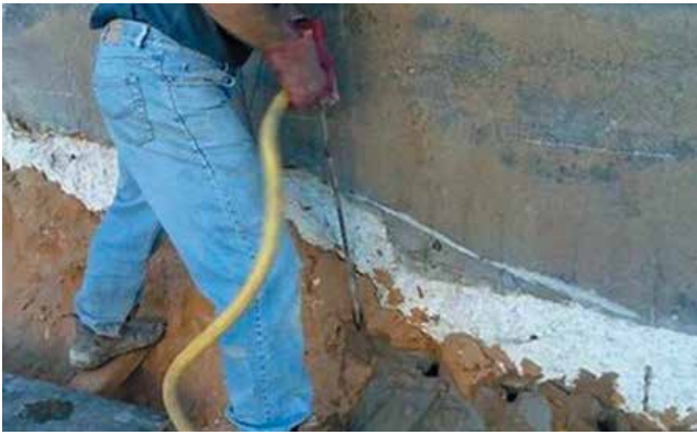
Figure 6. Bentonite injection on exterior side of foundation.
