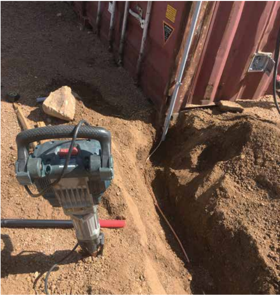
Figure 14. The soil density required a jackhammer to lay the proper grounding.
