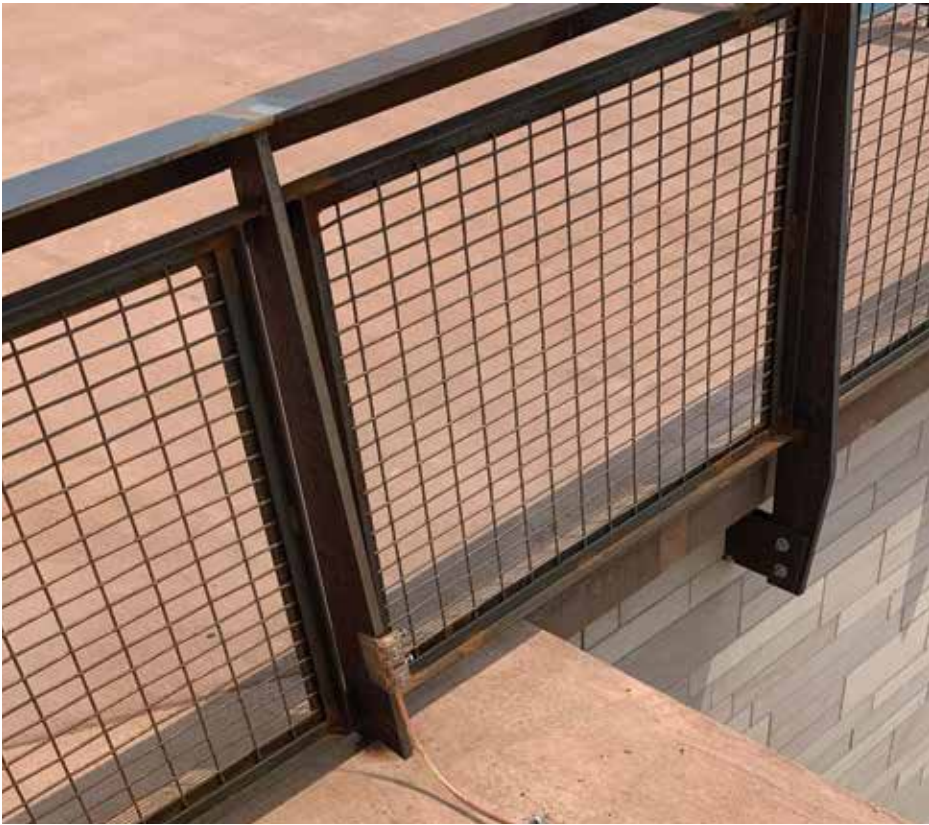
Figure 12. Permanent metal fabrications—including railings and roof gutters made from steel plate—used as strike termination devices and in lieu of conductor cables at the Summit Visitor Center at Pikes Peak in Colorado.
