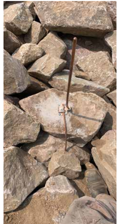
Figure 13. At the Summit Visitor Center at Pikes Peak in Colorado, copper components are used where they are adjacent to earth-toned materials—as seen in this boulder.
