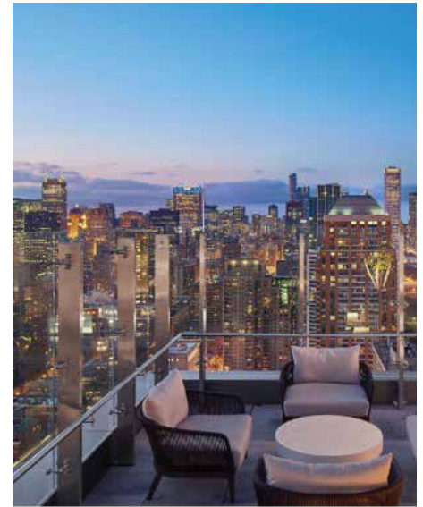
Figure 15. Early coordination on the assessment and design of this rooftop terrace enabled architects and engineers to uniquely use metal elements as part of the lightning protection system.
