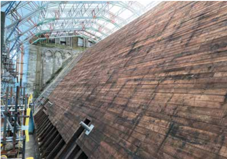
Figure 6. Copper removed, 1949 sheathing boards retained.
