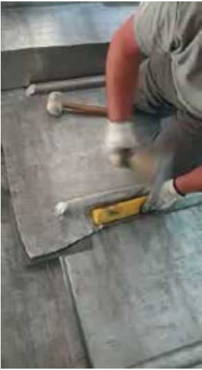
Figure 11. Lead dressed over timber batten rolls.
