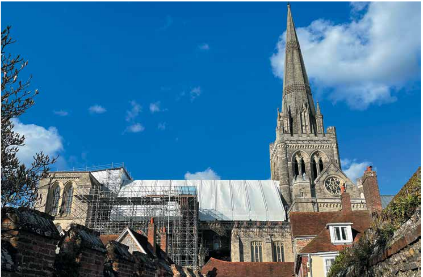
Figure 1. Extensive temporary works protecting the nave of Chichester Cathedral.
