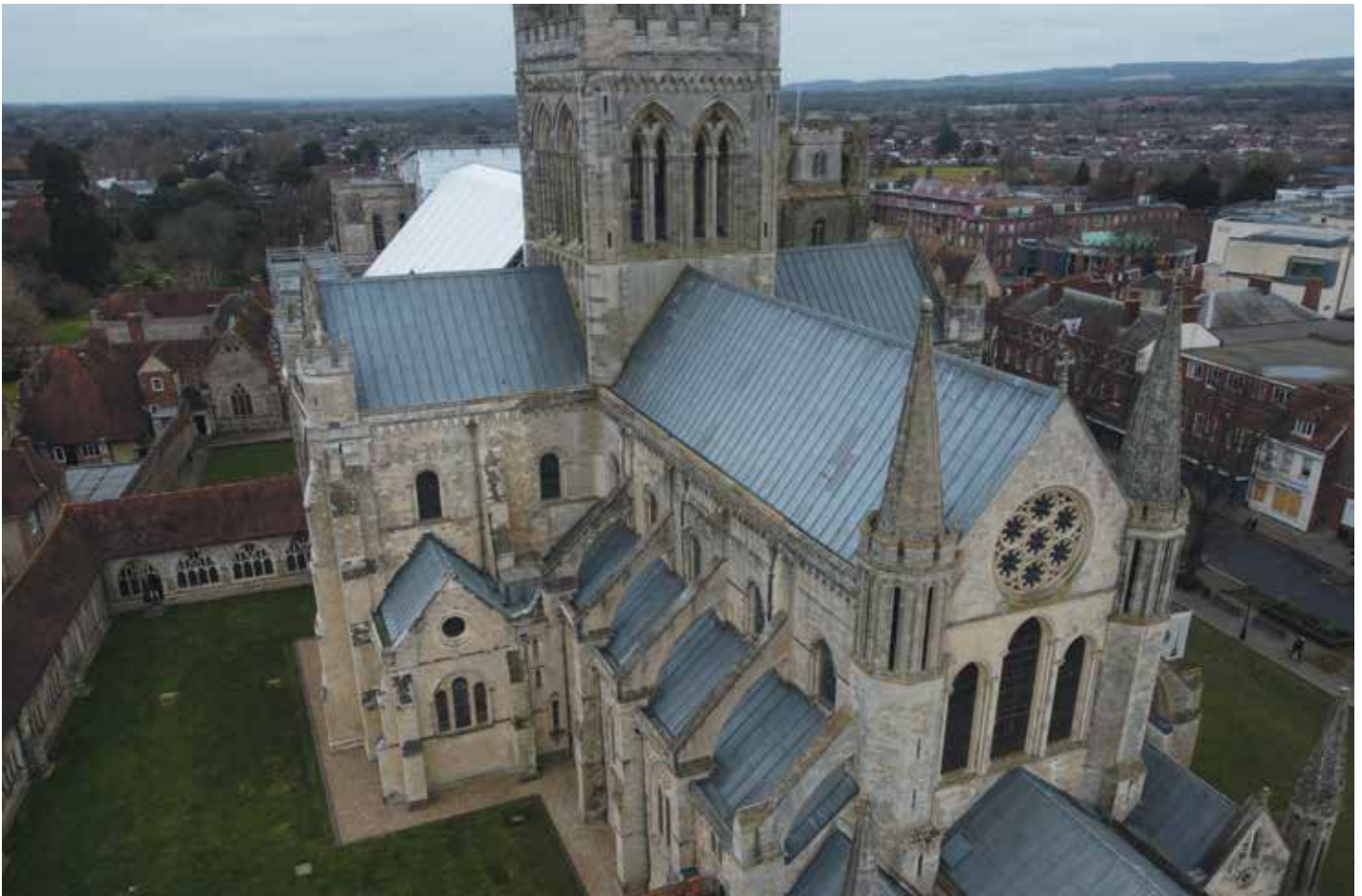
Figure 13. Completed lead roofing to chancel and transepts.
