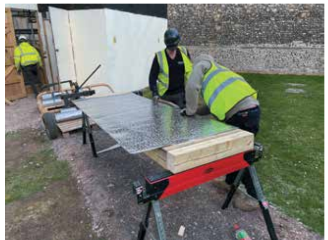
Figure 9. Lead cut to length and dressed on timber former.
