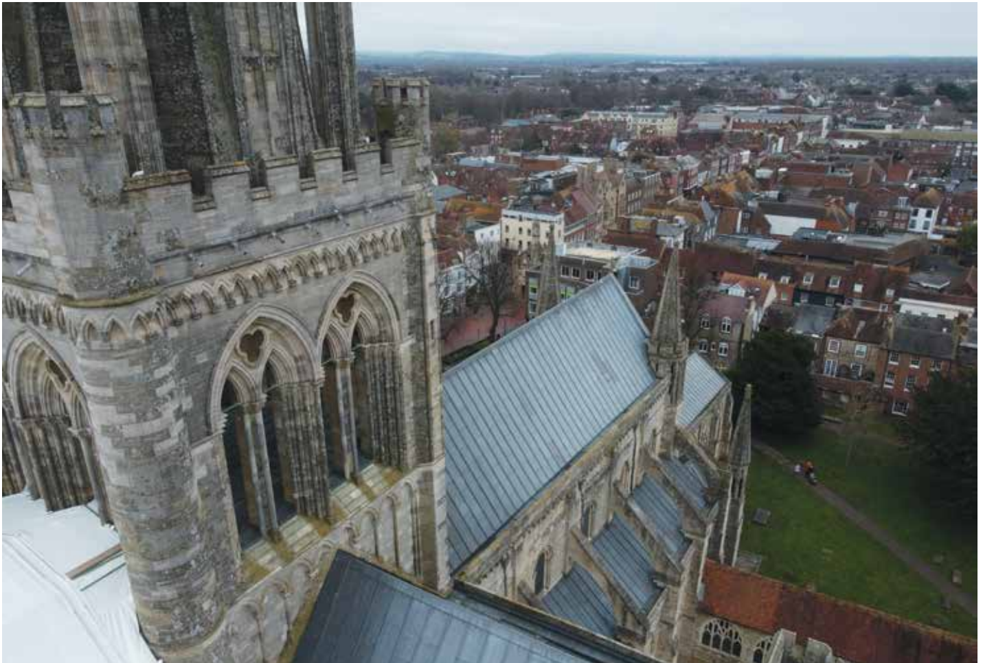
Figure 14. Completed lead roofing to chancel and transepts.
