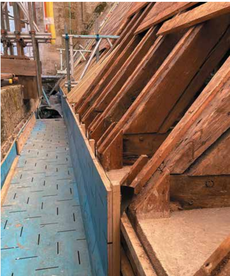
Figure 8. Plywood to support new gutter with ventilation slots.
