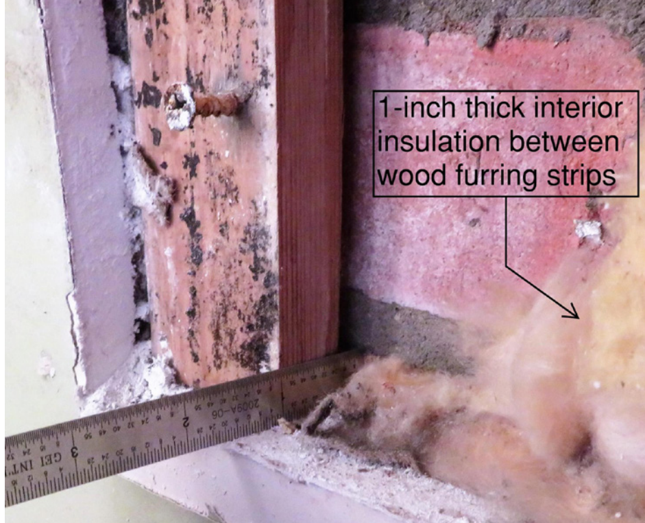
FIGURE 5. A thin layer of insulation provided on the interior side of a mass masonry wall.
