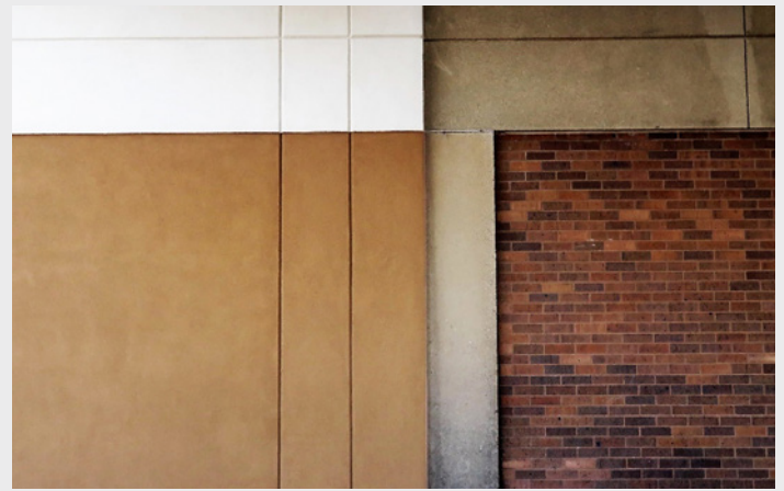
FIGURE 12. Completed overclad area of the EIFS adjacent to the existing masonry exterior wall.
