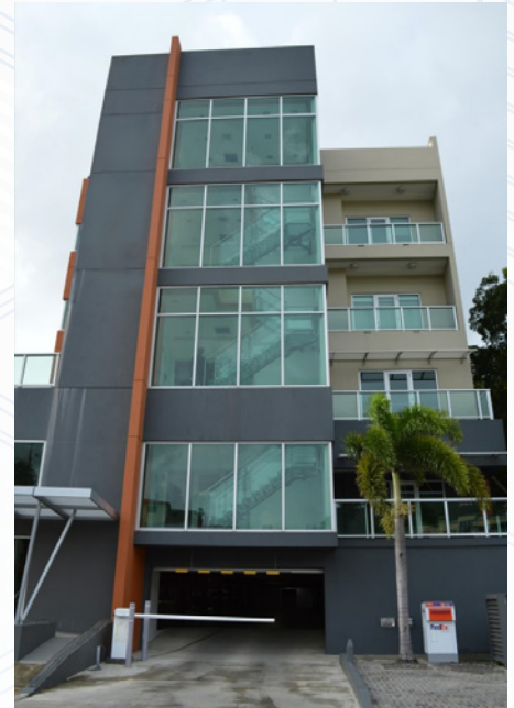
FIGURE 1. Overview of the Tortola Office Building.
