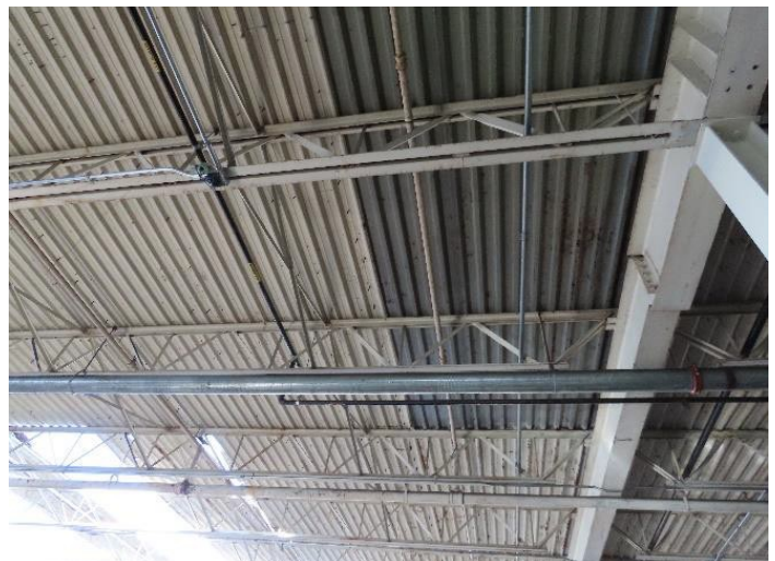
FIGURE 6. Replacement deck at right center.
