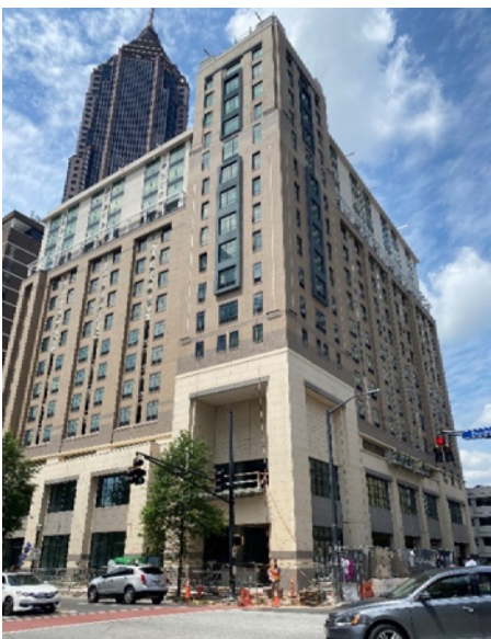
FIGURE 2. Completed building with prefabricated wall panels with a combination of EIFS and MVES.
