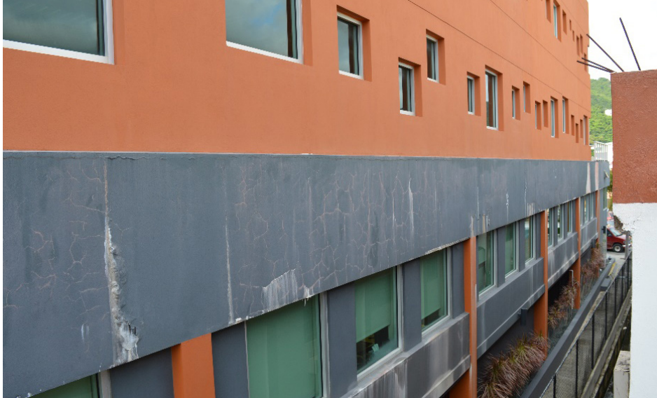
FIGURE 2. Concrete beam between the first and second floor where metal lath was used with stucco.
