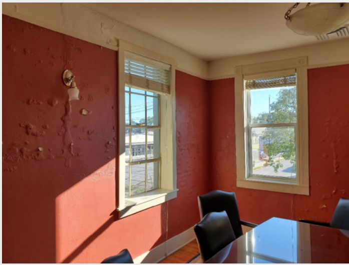
FIGURE 6. Representative view of unadhered pockets of interior coating with efflorescence behind unadhered coating.
