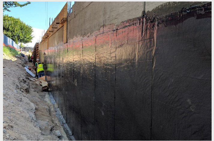
FIGURE 3. Installation of post-applied waterproofing membrane.
