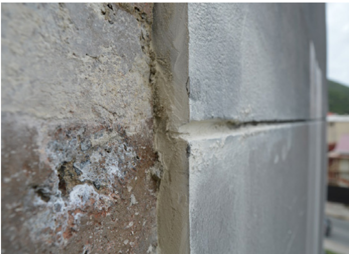
FIGURE 10. Destructive opening at a reveal of the stucco. No joint accessories were observed.
