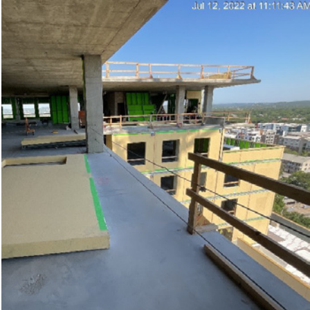
FIGURE 1. Prefabricated backup wall panels with framing, sheathing, and AWB. Some panels are installed into the wall, and panels on the floor await erection.
