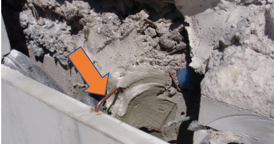
FIGURE 12. View of copper wire ties originally installed as lateral anchors in combination with mortar spots. Note that the wire tie is installed very close to the inside edge of the panel rather than centered.
