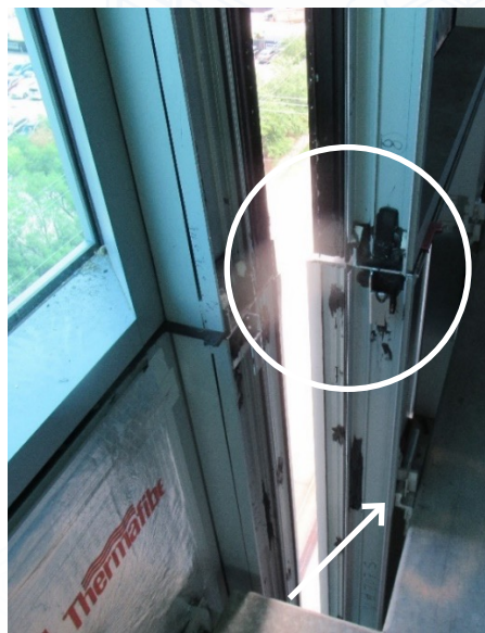
FIGURE 3. Unitized curtainwall in bypass application. Note unitized stack joint (circle) and curtainwall anchored to face of slab below (arrow).
