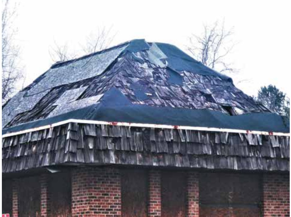
Figure 7. Roll-roofing placed across an old wood-shake roof.
