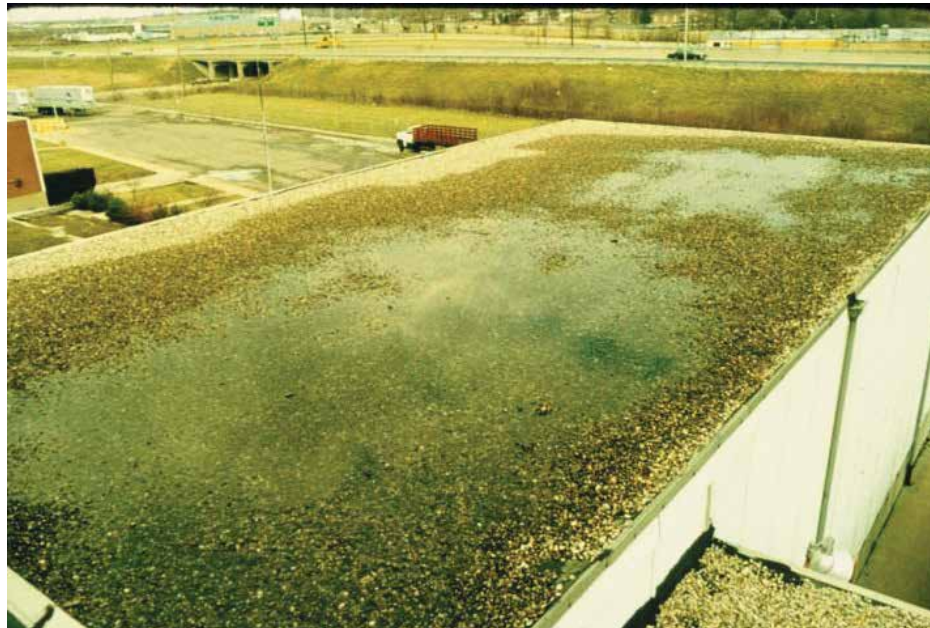
Figure 12. Insulated freezer panels can present genuine problems when over-roofing is needed. This midwestern freezer had experienced long-term creep and was subject to periodic drifting snow loads. As a result, it was perilously close to collapse when this photo was taken (circa 1984).
